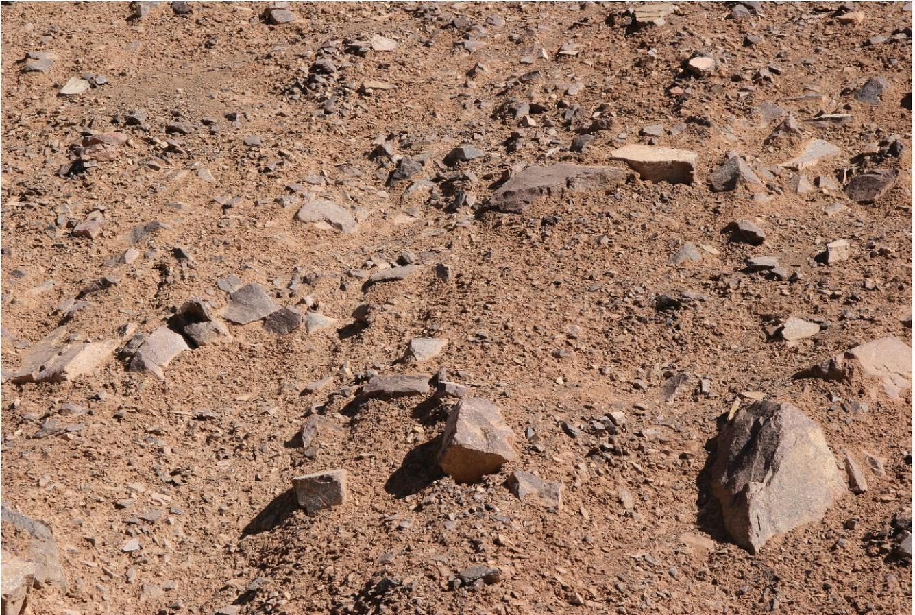
Figure 25. Close-up of the contaminated “dirty rock fill” exposed on lateral margins of the breach. The larger clasts are between 10 and 12 in. (25.4 to 30.5 cm) in diameter.
