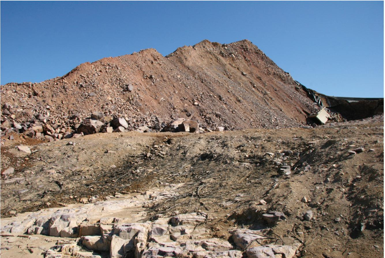
Figure 31. Residual soils, including tree roots, were observed in-place beneath the “plinth area” in the northwest corner of the Upper Reservoir, where a portion of the embankment was founded on as much as 10 to 16 ft (3 to 4.9 m) of residuum and a thin layer of rock fill.
