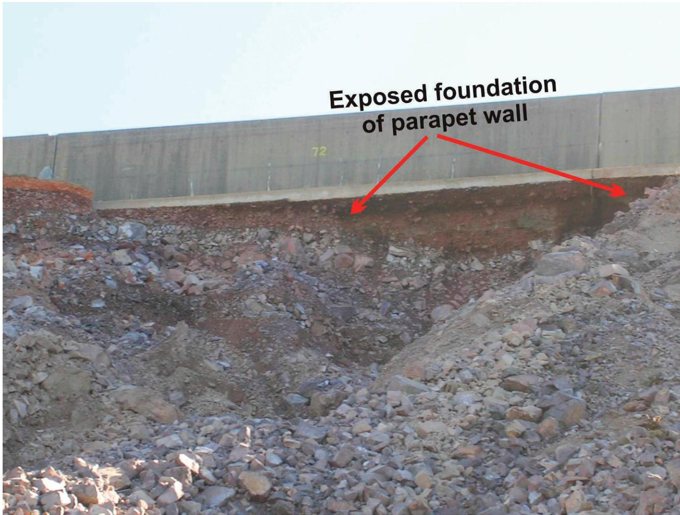
Figure 13. This photo, taken below panels 71–72, shows the plunge pool excavated beneath the parapet wall, which completely undermined the wall and is the basis for Figure 16 (photo courtesy of David J. Hoffman).
