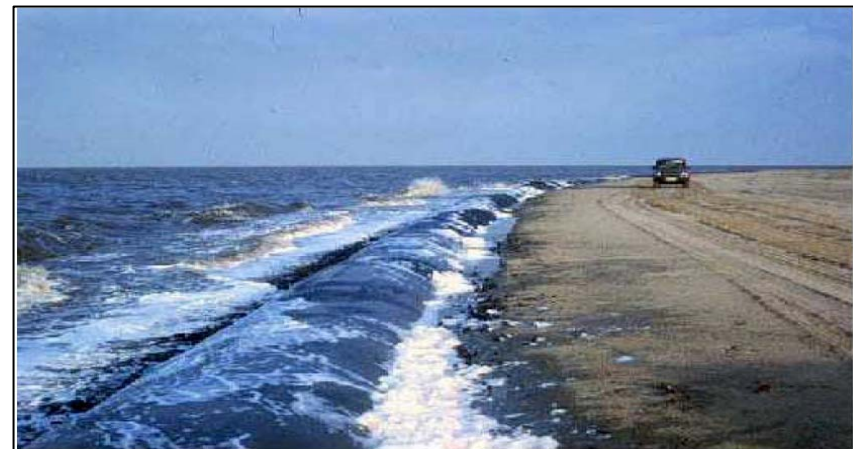
Figure 3. Photograph of Geotube™ Dike with Dredged Fill behind Geotube™ in the Netherlands
