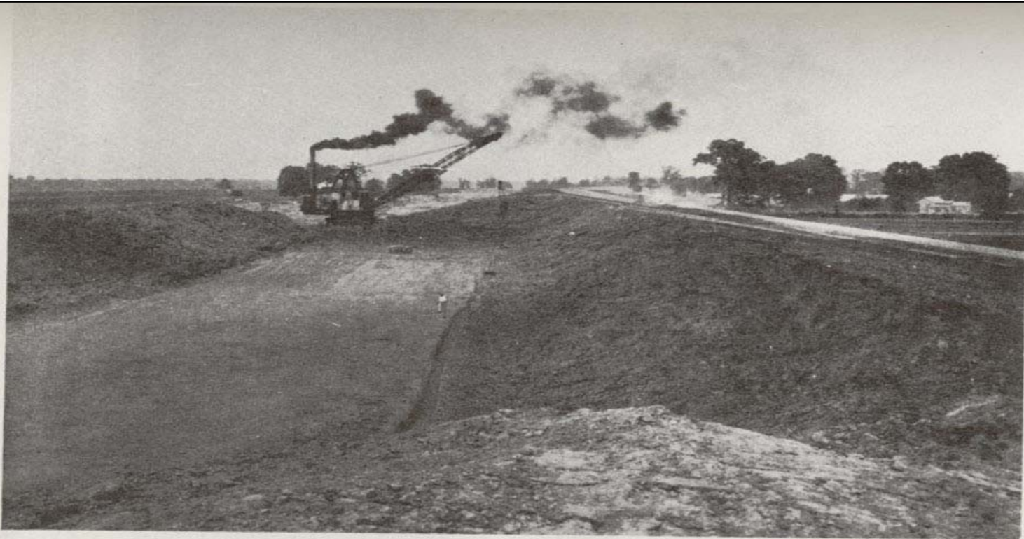
LEVEE CONSTRUCTION BY DRAGLINE Morrison-Picayuneville Levee about 25 miles below New Orleans. June 15, 1931
