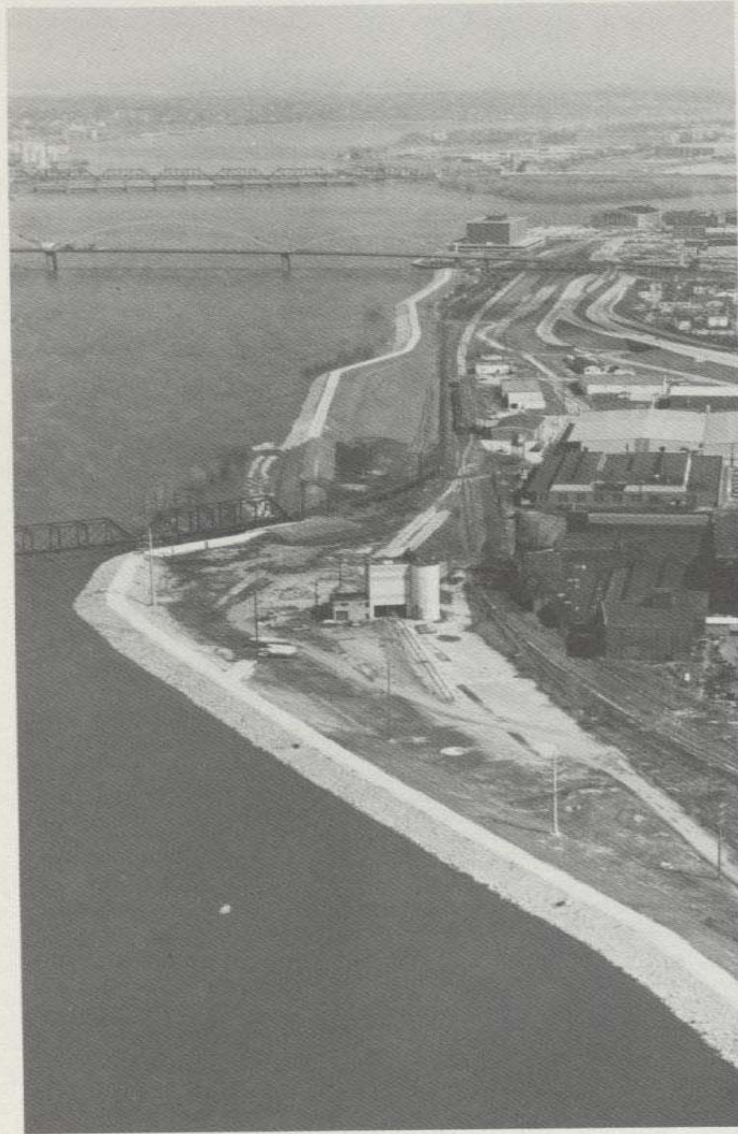
FIG. 72. The newly completed Rock Island levee kept Rock Island dry during the 1973 flood.
