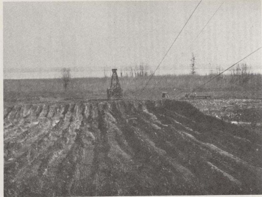
LEVEE CONSTRUCTION BY TOWER MACHINE
