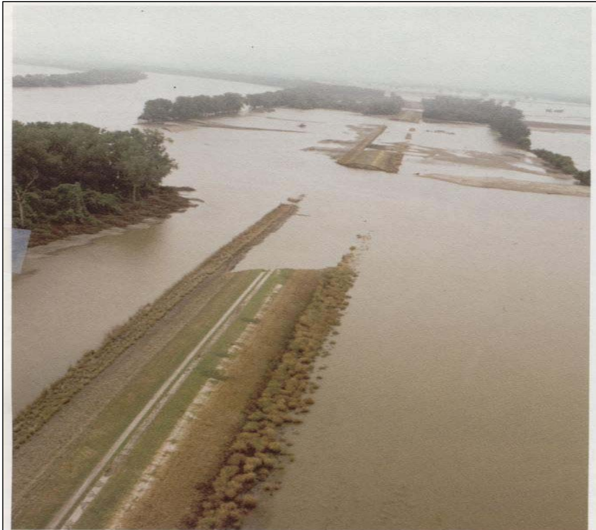
Federal Levee L246 at RM 241 on the Missouri River.
