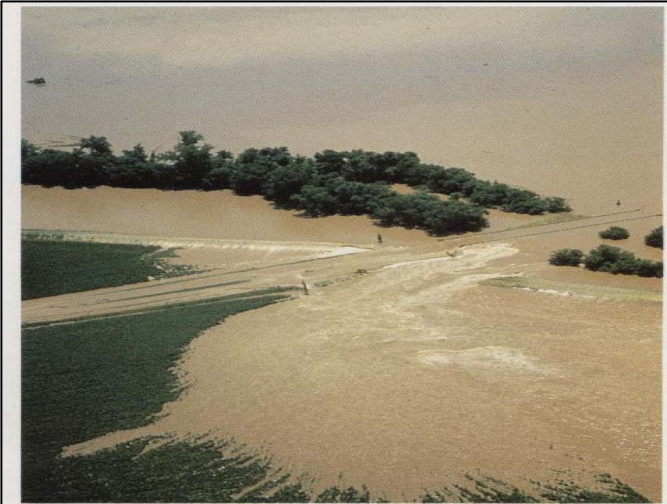
The Missouri River defeated this levee near Boonville, Missouri.
