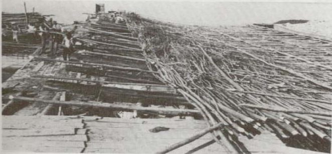
Rock is piled on floating mattress for ballast
