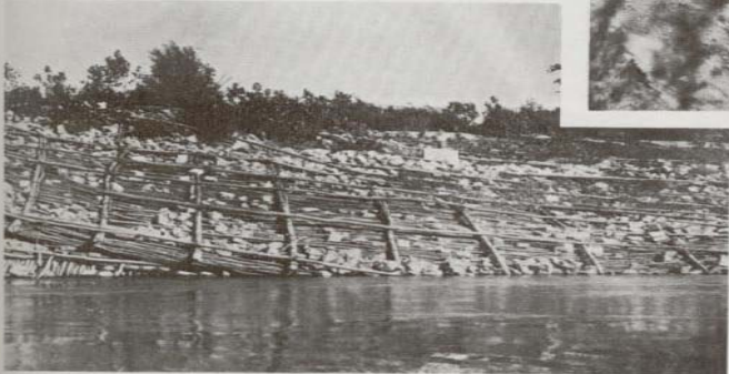
Mat in place, remainder of willows are below water level
