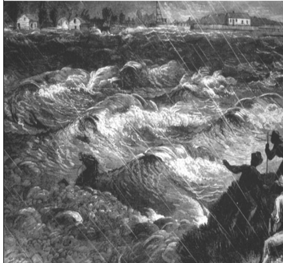
Levee crevasse at Bonnet Carré, Louisiana.
