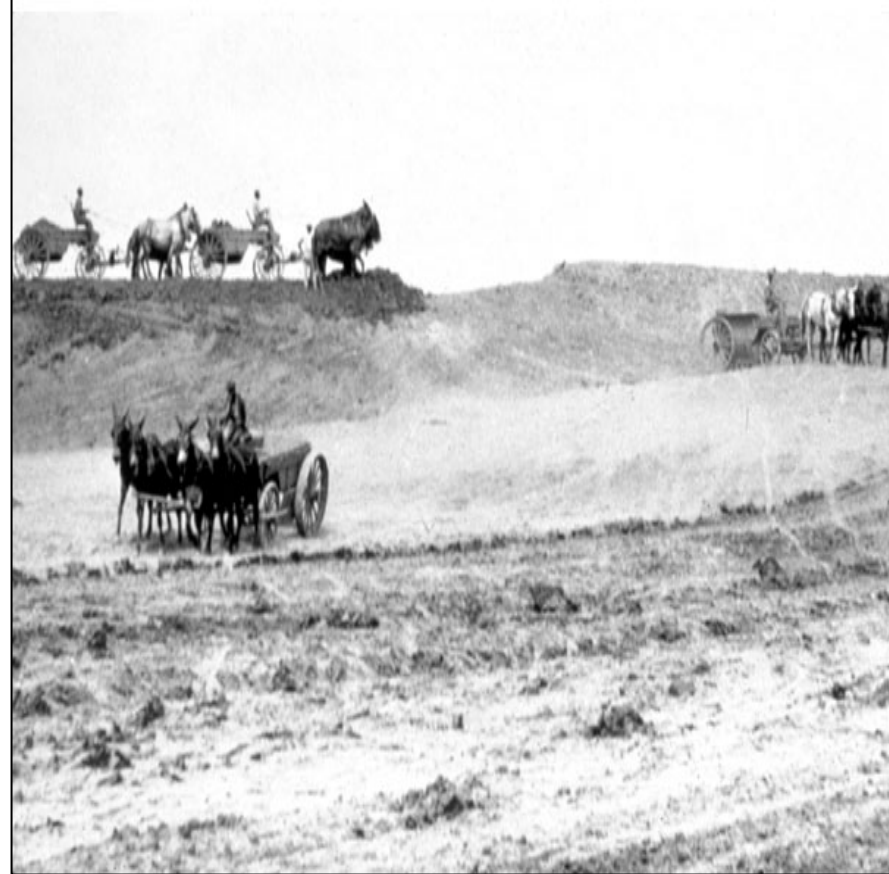
Mules and wagons are used to construct levees in the St. Francis Levee District in 1909.
