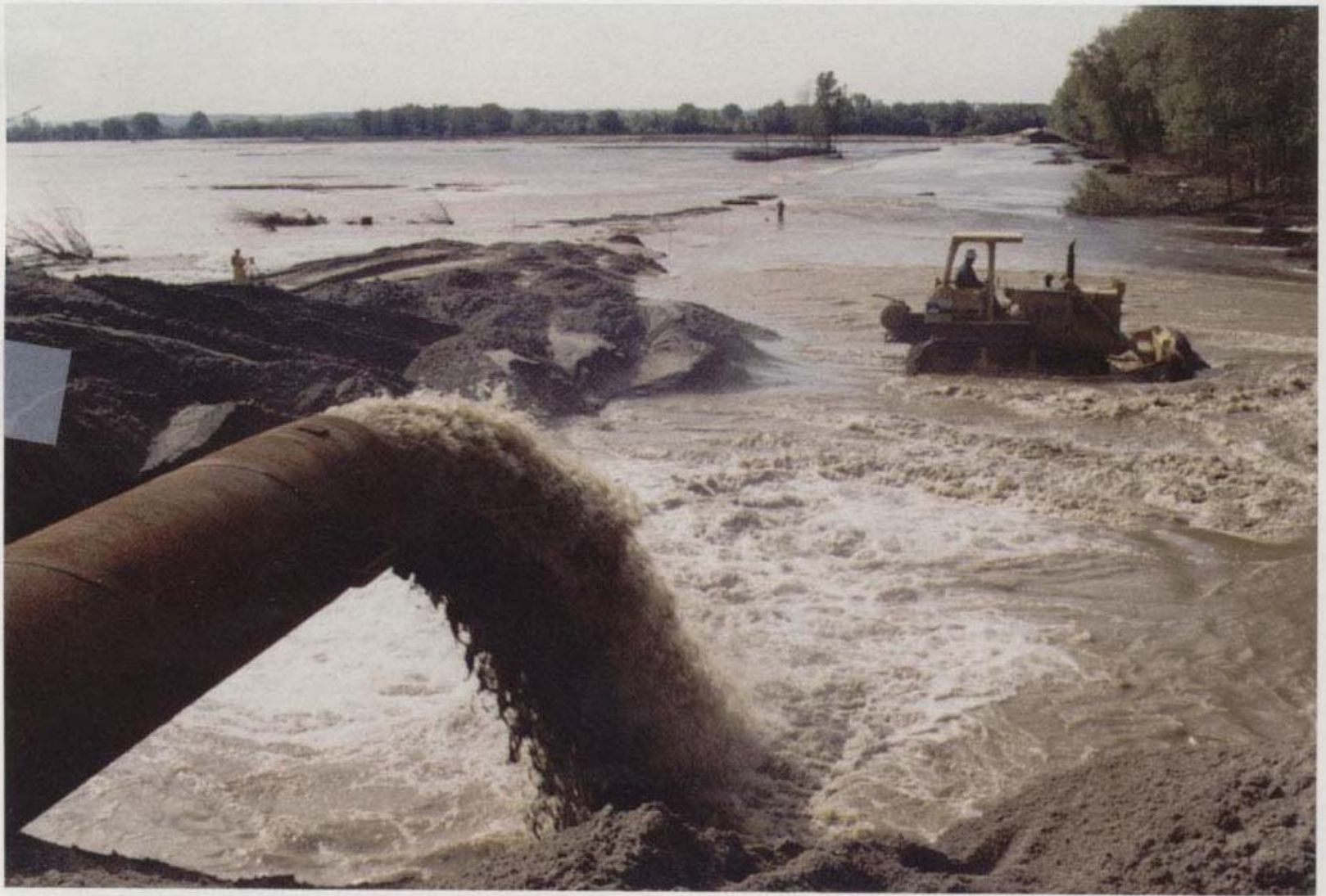
Hydraulic dredges repairing the damaged Sny levee.
