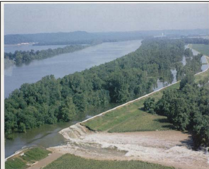
Nutwood Levee break on the Illinois River.
