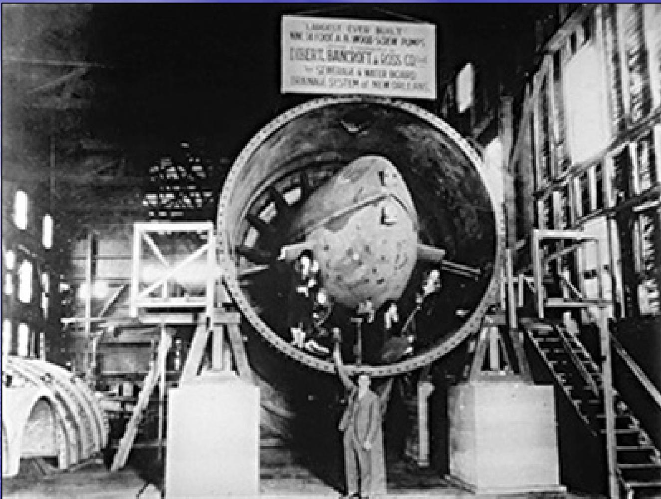
**A. Baldwin Wood** was a young S&WB engineer who designed the enormous screw pumps, 12 to 14 feet in diameter, which run on 25 Hz electric power using 20 ft diameter dynamos. The City began by installing 11 Wood pumps in **1915** for a cost of \$159K. These replaced the old steam powered paddle wheel pumps.
