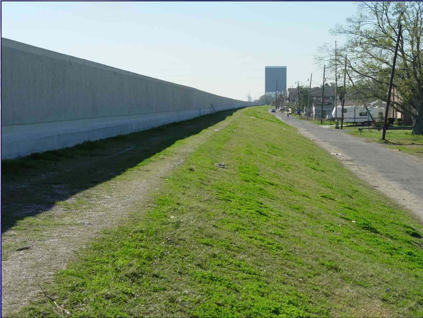
**Flood Walls were constructed on the crowns of drainage canals and the Inner Harbor Navigation Canal to accommodate functionality during high storm surges. The walls in the Lakeview and Gentilly Districts topped out at +14 ft above MGL.**
