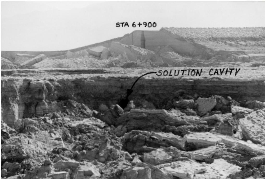
**Figure 10** – 2.5 km of a 25 m high dike constructed for potash extraction failed during its initial filling in March 2000. The Lisan formation formed the dike foundation, on ground reclaimed in 1988 as the Dead Sea dropped. Several solution cavities were noted at 2 m depth, below an algal aragonite horizon. Photo by author.
