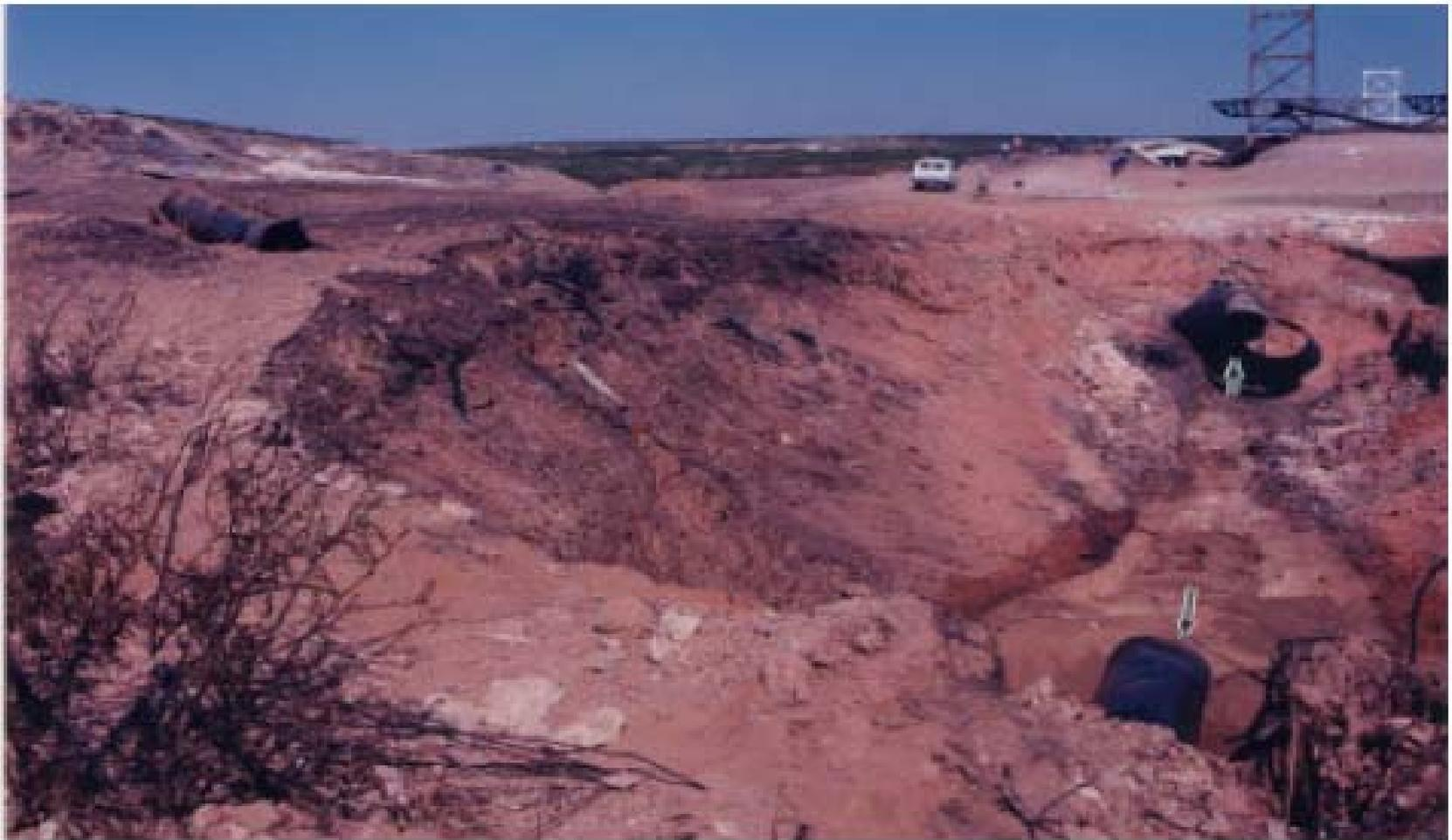
**Looking west at a portion of the blast crater. Four sections of pipe (comprising 49 lineal feet) between the arrows were ejected from the crater. A 22 ft long segment was recovered 270 feet from the crater.**
