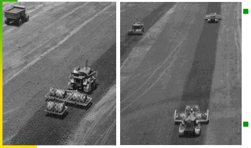
The two Bouquet Canyon zoned fill embankments were constructed by the Los Angeles Department of Water & Power between 1932-34 to replace the St. Francis concrete dam, which failed in 1928.
