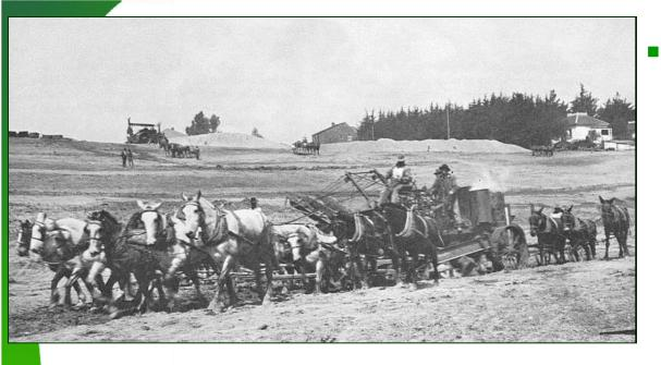
Above left: 10-horse team pulling an elevating grader to load hopper dumping wagons during construction of the **Central Reservoir** for the People's Water Co. in Oakland, California in 1909. Note old Buffalo-Springfield steam roller
