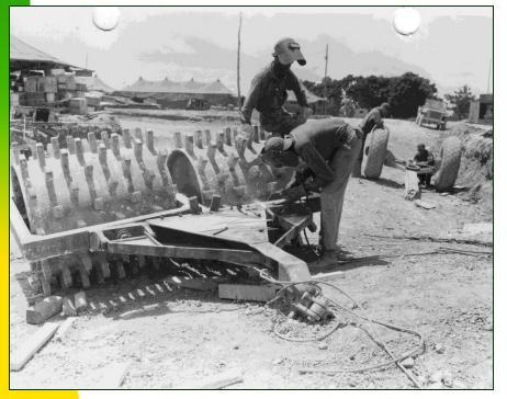
**During the Second World War** (1941-45) square spiked rollers were mass produced because the teeth could be fabricated easily.
