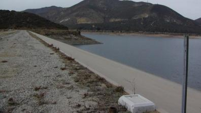
The Bouquet Canyon embankments were carefully constructed and monitored over the next 20 years. They ushered in a new era of mechanically compacted embankments. Their 3:1 upstream faces were re-lined with concrete slabs in 1981.
