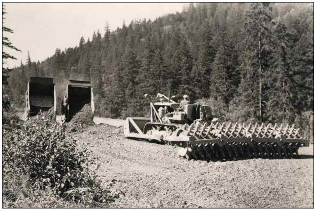
The 1930s and 40s witnessed the rapid development of mechanical compaction of soils, using increasingly larger equipment, often fashioned by contractors. This view shows quadruple 3-ft diameter 5,000 lb rollers, typical of highways work by 1940, just before the Second World War.
