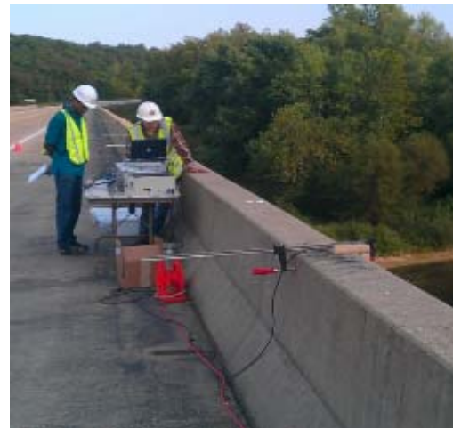
(b) Over Bridge Deck
