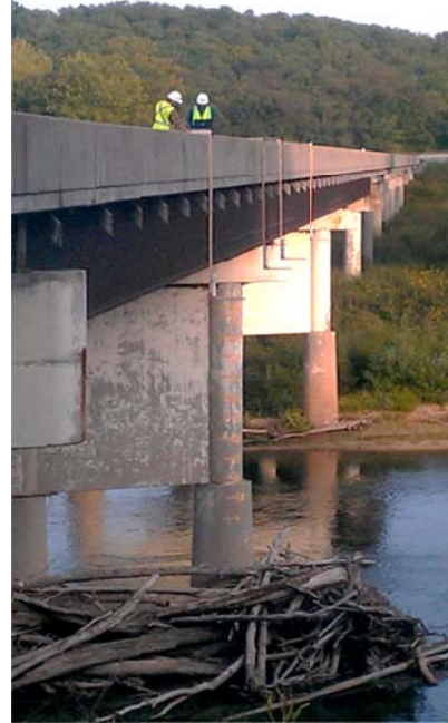
(b) Four Antenna Holders Hung on Bridge Rail
