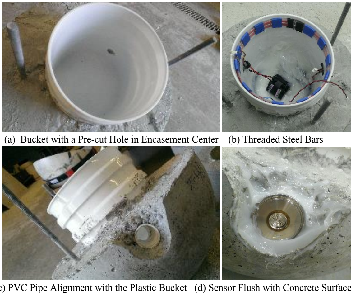
Figure 4.40 Installation of Pressure Sensor in a Smart Rock
