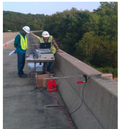
(c) Base station at bridge deck
