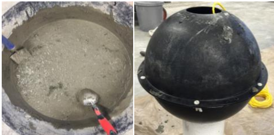
(a) Prepare Fiber Reinforced Concrete (b) Place an APUS into Concrete and Mold
