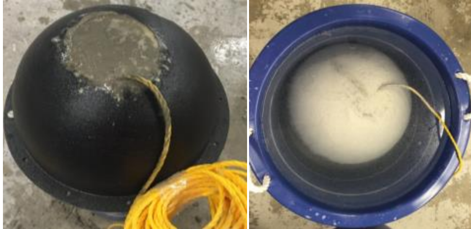
(c) Fill the Mold with Concrete (d) Cure the Concrete Encasement in Water for 14 Days Figure 4 Fabrication of Concrete Encasement
