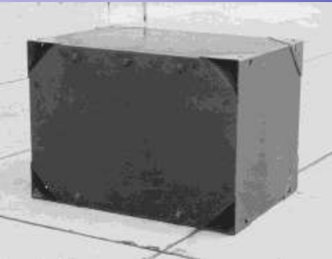
The standard Type 6 steel pontoon boxes were 5 ft x 7 ft x 5 ft.
