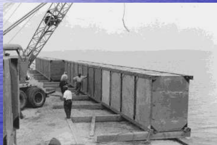
“Pontoon strings” were fabricated by employing steel angle stiffeners along each corner.
