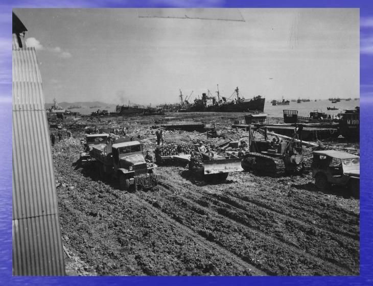
The soft organic soils lying within poorly drained coastal mangrove swamps had to be filled in and the roads paved with free-draining coral.
