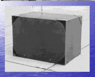
The standard Type 6 pontoon boxes were 5 ft x 7 ft x 5 ft. These were shipped flat, then assembled in-theater. Tapered Type 7 pontoons were attached to the ends of pontoon barges, to aid their navigation through open water.
