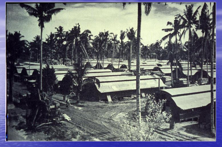
Late model tropical Quonset 20 huts with upturned side walls at the Philippine Sea Frontier headquarters at Tolosa on Leyte, constructed by the 61<sup>st</sup> Seabees in January 1945. The entire hut was fitted with screens to promote cross ventilation. These modifications came about as a matter of necessity and comfort, operating in extreme heat and humidity.
