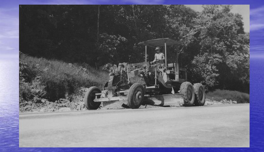
The Seabees used every variant of the road grader manufactured in the United States. Graders were essential to the upkeep and maintenance of the road network. Note protective hood added in the field.
