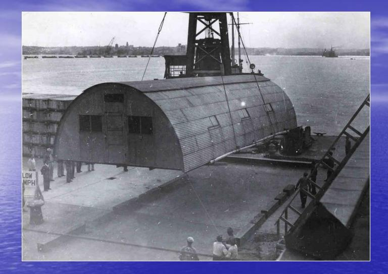
Mobile crane lifting an assembled Quonset 20 to a newly poured foundation, while constructing a base in occupied Japan in early 1946.
