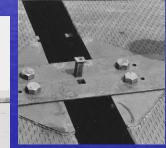
Link pin being driven into top angles connecting adjacent strings of pontoons
