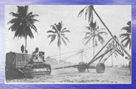
Men of the 62nd Naval Construction Battalion filling in erosion ravines caused by a tropical storm in July 1945 on Iwo Jima A Seabee uses a special jig frame used to uproot coconut palm trees.
