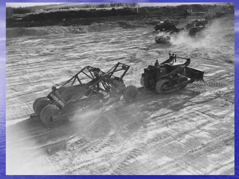
Most airfields projects were completed in 14 days. The bulk of this work involved laying down high-quality engineered fill and compacting it.
