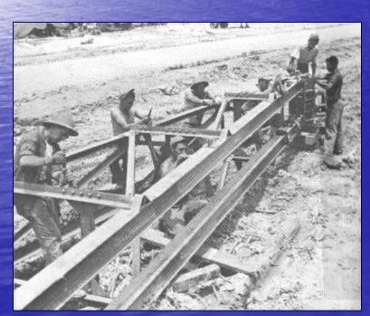
Men from the 7<sup>th</sup> Battalion assemble the tower of a pile driver for use in construction work on Okinawa.
