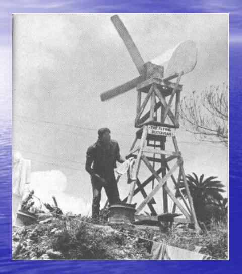
**A Seabee on a Pacific** island loads his "cumshaw" washing machine. The clothes go into the drum, which is then placed on the plank under the tower. As the windmill spins, the plunger — an inverted funnel-goes up and down to slosh the clothes about in the water.
