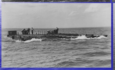
Load tests on two self-propelled 3 x 12 50ton barges, their maximum capacity 6 x 12 pontoon seaplane barge, carrying a Martin PBM Mariner patrol bomber
