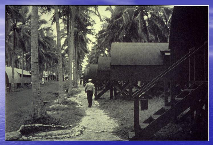
Prefabrication of Quonset frames was a necessity in those islands subject to severe flooding during the summer monsoon season. This shows completed huts on elevated frames, to keep their contents dry during seasonal inundation of the local flood plain. This shows Naval Hospital No. 3 at Espiritu Santo.
