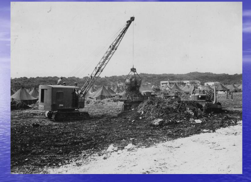
The first two days of airfield construction typically involved extensive grubbing of vegetation
