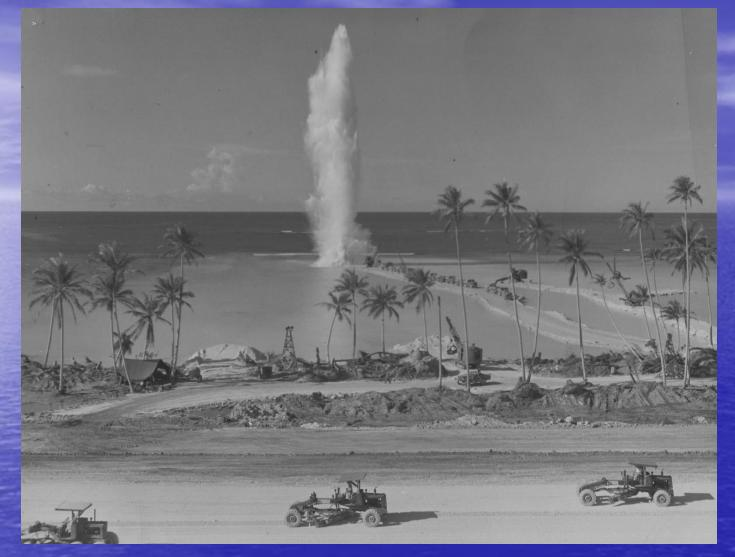
Setting off demo charges in coral reef to allow collection of live coral for paving airstrips
