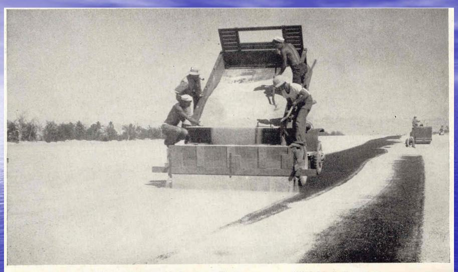
5. Surfacing with finely crushed coral - twelfth day.
