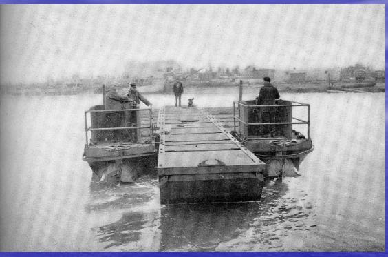
7-12-7 pontooon tugboat (shown above and at bottom left) was assembled from Type 6 and Type 7 steel pontoons, with two 1-AT marine tractor motors for propulsion
