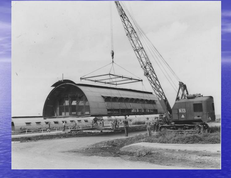
Q20 huts were routinely assembled on jigs and then moved by crane onto their foundations. Note lifting frame used to spread the four cables.
