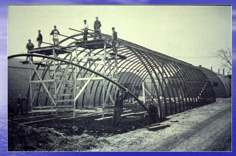
The larger Elephant Huts were usually assembled directly upon on gravel pads and/or concrete floors of their building pads, as shown here. Note temporary scaffolding.
