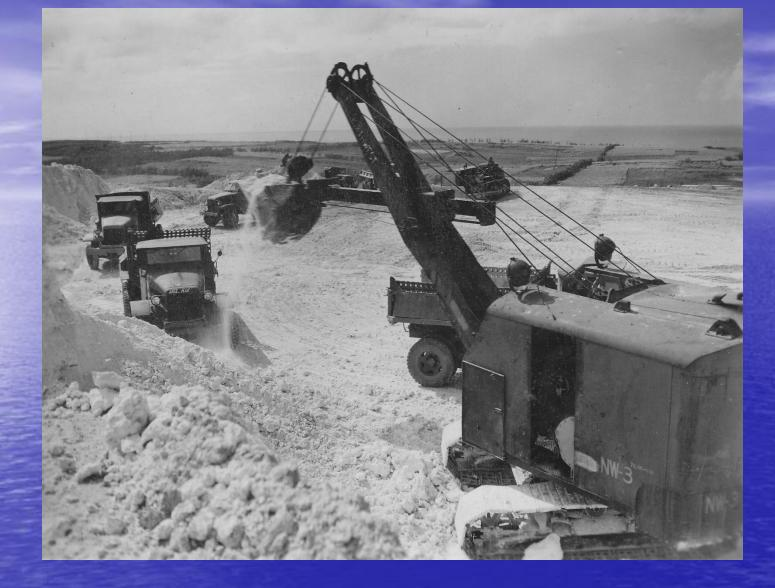
The essential first step in grading any airfield was to set up a quarry and crushing/classification. This shows a runway quarry on Tinian.
