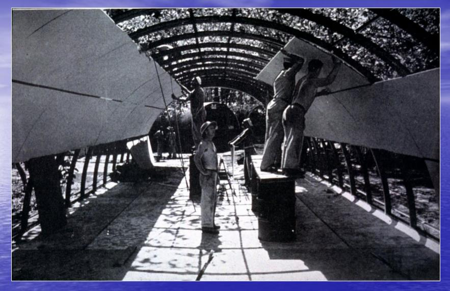
Interior Masonite panels were nailed to the inside of the steel frame ribs, as shown here, somewhere in the South Pacific. Metal splines were then installed between the sheets. Note plywood floor, already in-place.
