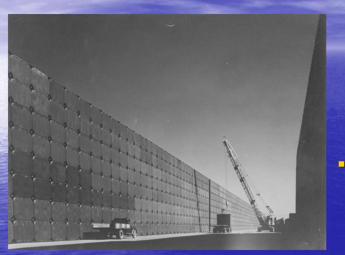
Dozens of subcontractors produced the ubiquitous Type 6 steel pontoons shown here at Port Hueneme, which were 5 x 7 x 5 ft Each pontoon weighed 2000 lbs and were shipped flat, then assembled onsite
