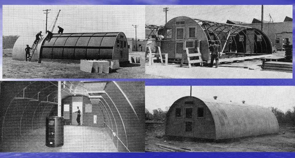
Details of the original Fuller-built 16'  $\times$  36' Quonset Huts, assembled at West Davisville in the summer of 1941. The American hut employed masonite interior walls with a galvanized steel shell, and the gap filled with insulation.
