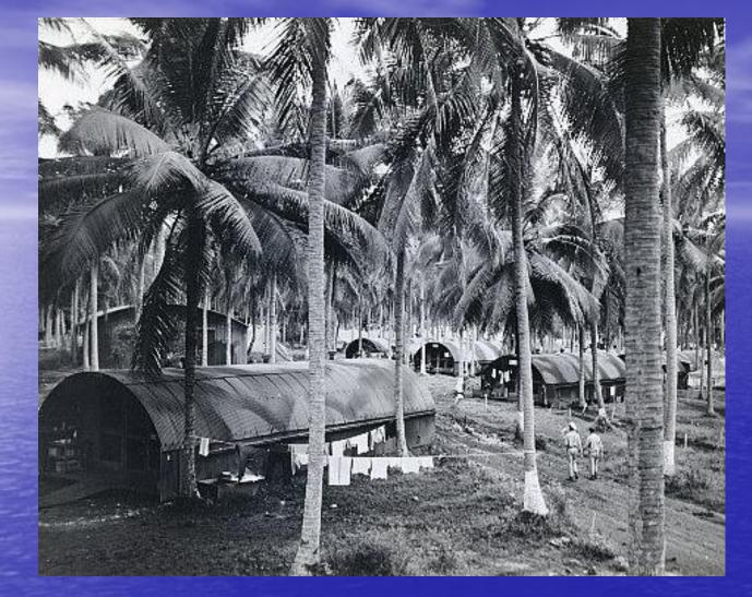
In late 1942 the standard Q20 hut was re-designed with straight sides to better utilize floor space, but these required additional cargo space, so the Navy reverted to the hemispherical design.
