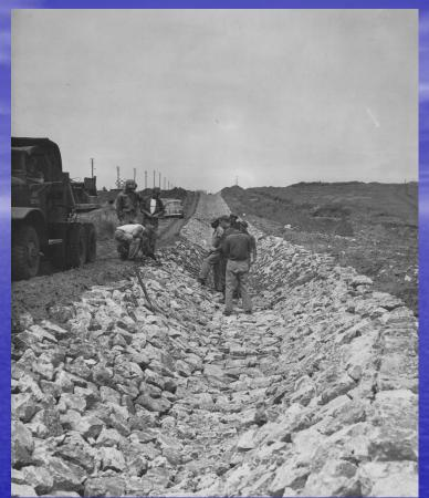
Filling, compaction, and drainage were the essential elements of highway construction
