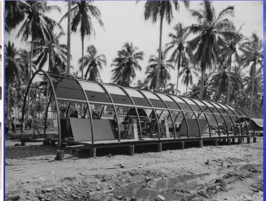
The assembly instructions directed that the Masonite lining be installed first, followed by the wood fiber insulation, then by the exterior corrugated steel sheathing. Image at right shows window and door frames/dormers on a standard 20-by-48 ft Quonset Hut, produced by Stran-Steel.
