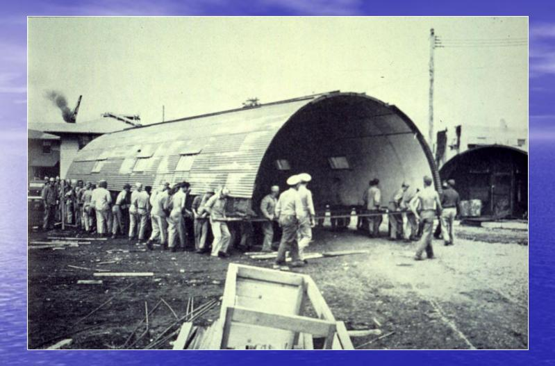
Several dozen Seabees of NCB 90 man-handle a 20 by 48 Quonset Hut on Iwo Jima using steel stretchers with pipe handles, moving it to a new location. An empty hut weighed about 7000 lbs
