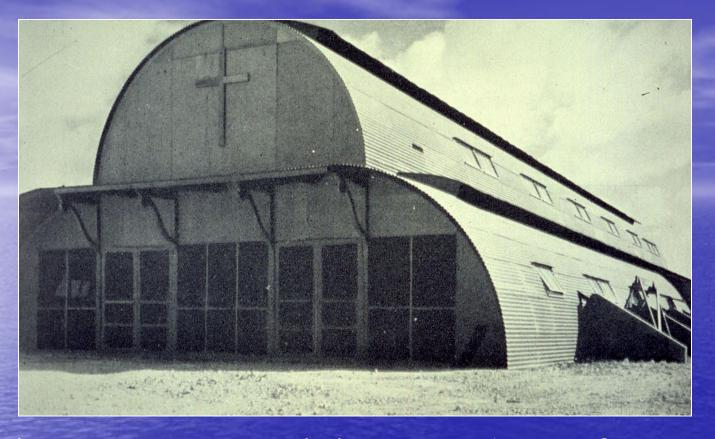
This shows an improvised design combining four standard Q20 Quonset Hut kits to fashion a non-standard base chapel, built by the 117<sup>th</sup> Seabees on Saipan. Note concrete thrust blocks along the right side, to accommodate the loads of the upper hemisphere shell.
