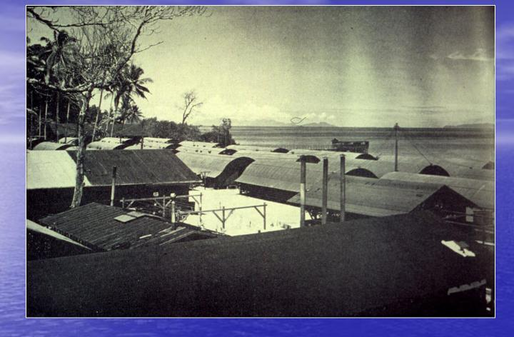
From mid-1943 onward, virtually all of the standard Quonset 20s were modified during construction with open, upturned sides to make them more bearable in tropical climates. This shows the living quarters at Carter City on Florida Island in the Solomons. Frame structures in foreground are the base laundry and one of the power plants.
