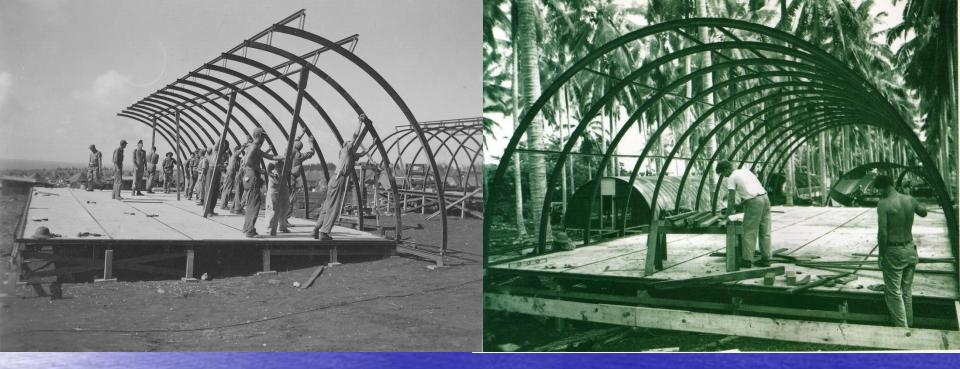
Quonset Huts were known for quick erection of arched frame ribs and connecting purlins. This shows a hut being assembled on a jig, or erection platform by 33<sup>rd</sup> Naval Construction Battalion in the Russell Islands in Nov. 1943. The exterior sheathing was nailed to the frames and the purlins. After assembly of the frame and exterior sheathing, the unit was moved to its pad (note completed shells in background).
