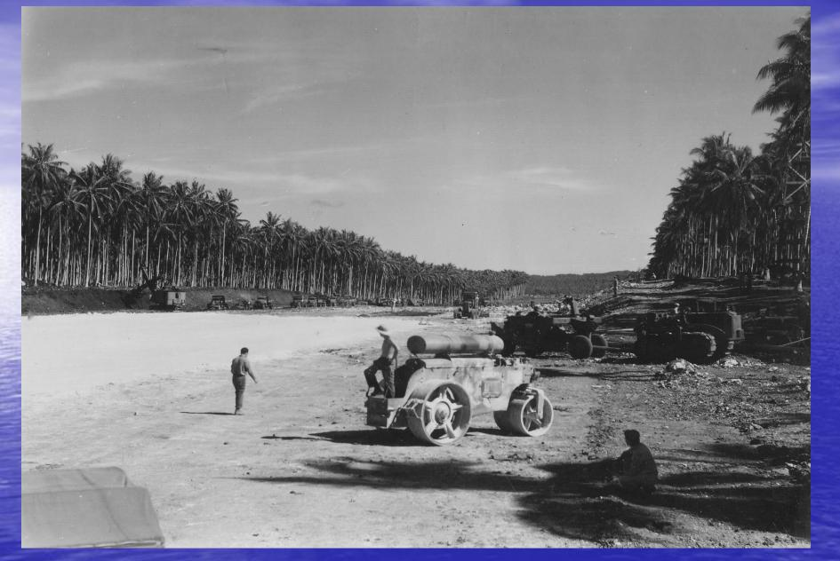
Paving stone for the main runway begins to be rolled from one end to the other by Day 8.
