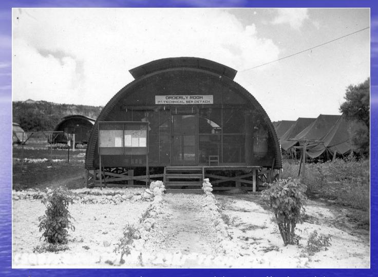
**Tropical Quonset 20** with its raised 'umbrella hood,' occupied by elements of the 509<sup>th</sup> Composite Group on Tinian in 1945. Tropical Quonsets employed screened end walls, raised roofs, and additional vent flaps along their sides to promote better air circulation. Note elevation of floor in this example, well above the ground. This enhanced better cooling as well.
