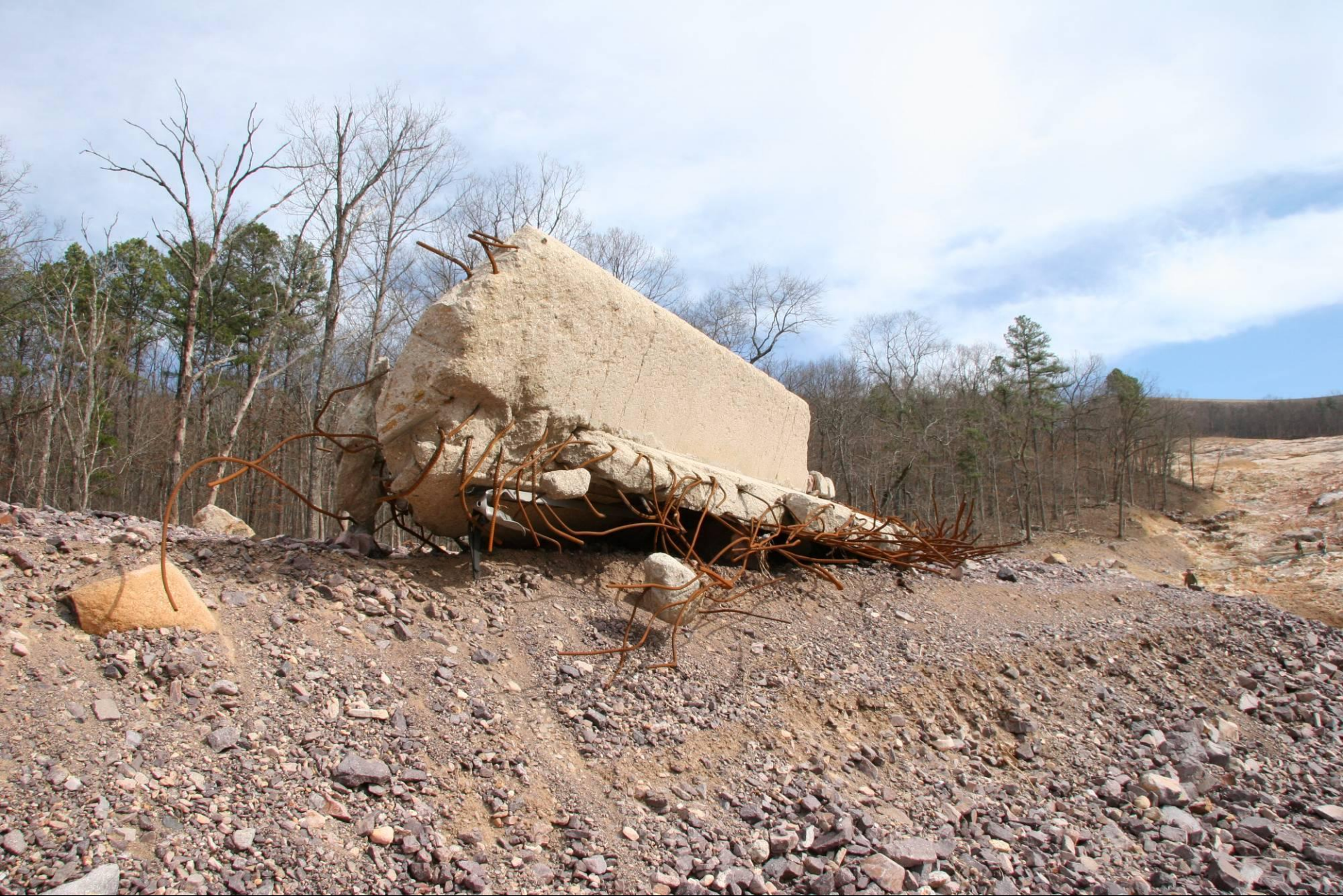
Huge pieces of rock and concrete were carried downslope by the turbid flow. A large section of a concrete wall panel is shown here.
