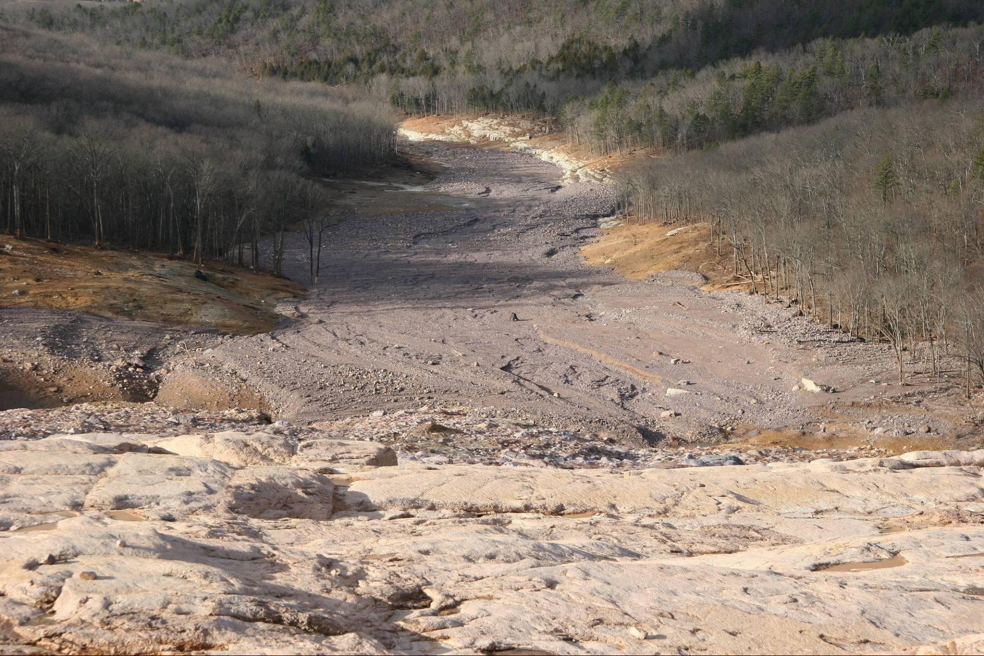
Lower portion of the scour channel and precipitous drop, immediately below the reservoir. Note demarcation between bedrock and gravels.
