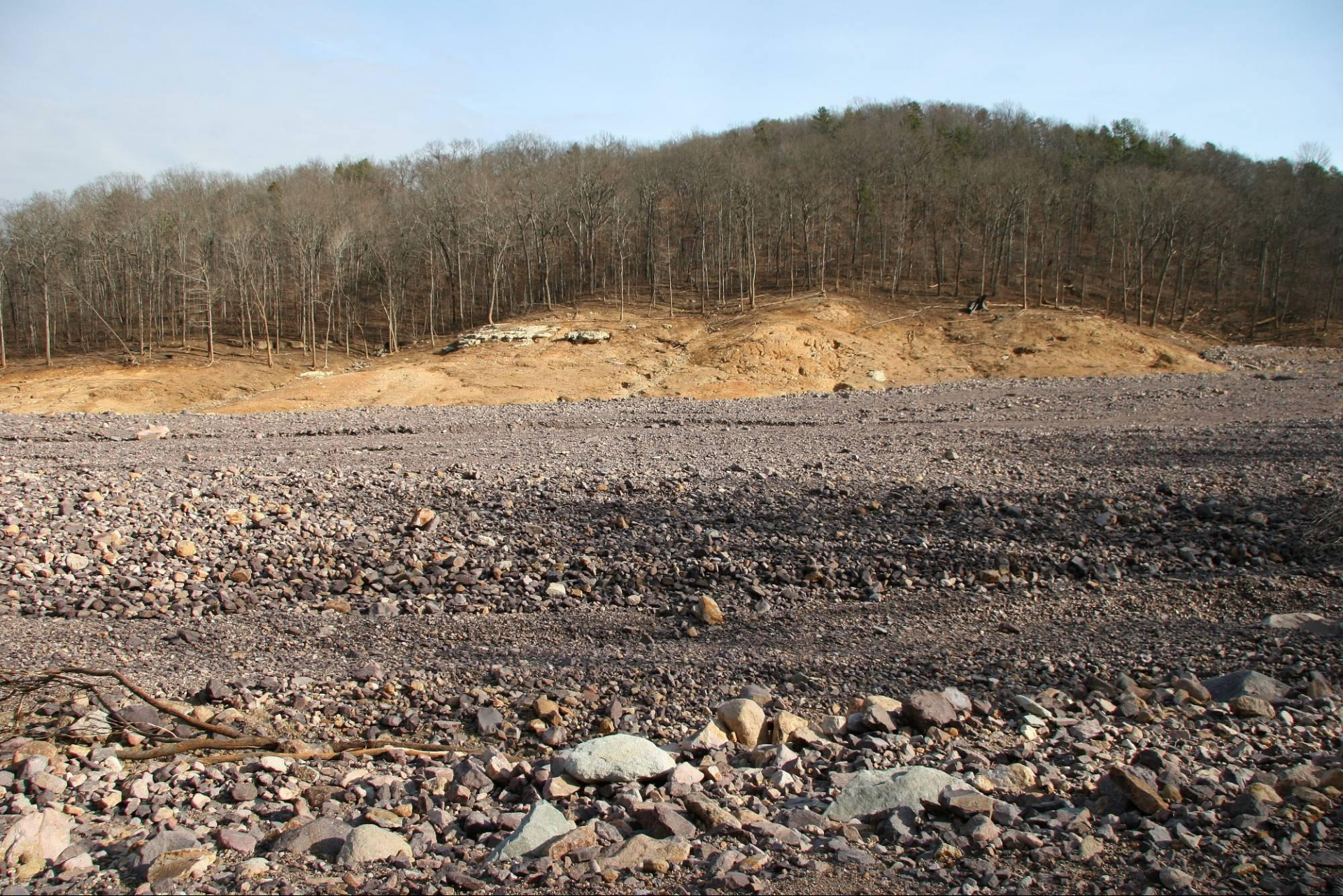
Reworked boulders, cobbles, and gravels fill the lower portion of the scour channel, along with twisted remnants of concrete and rebar.
