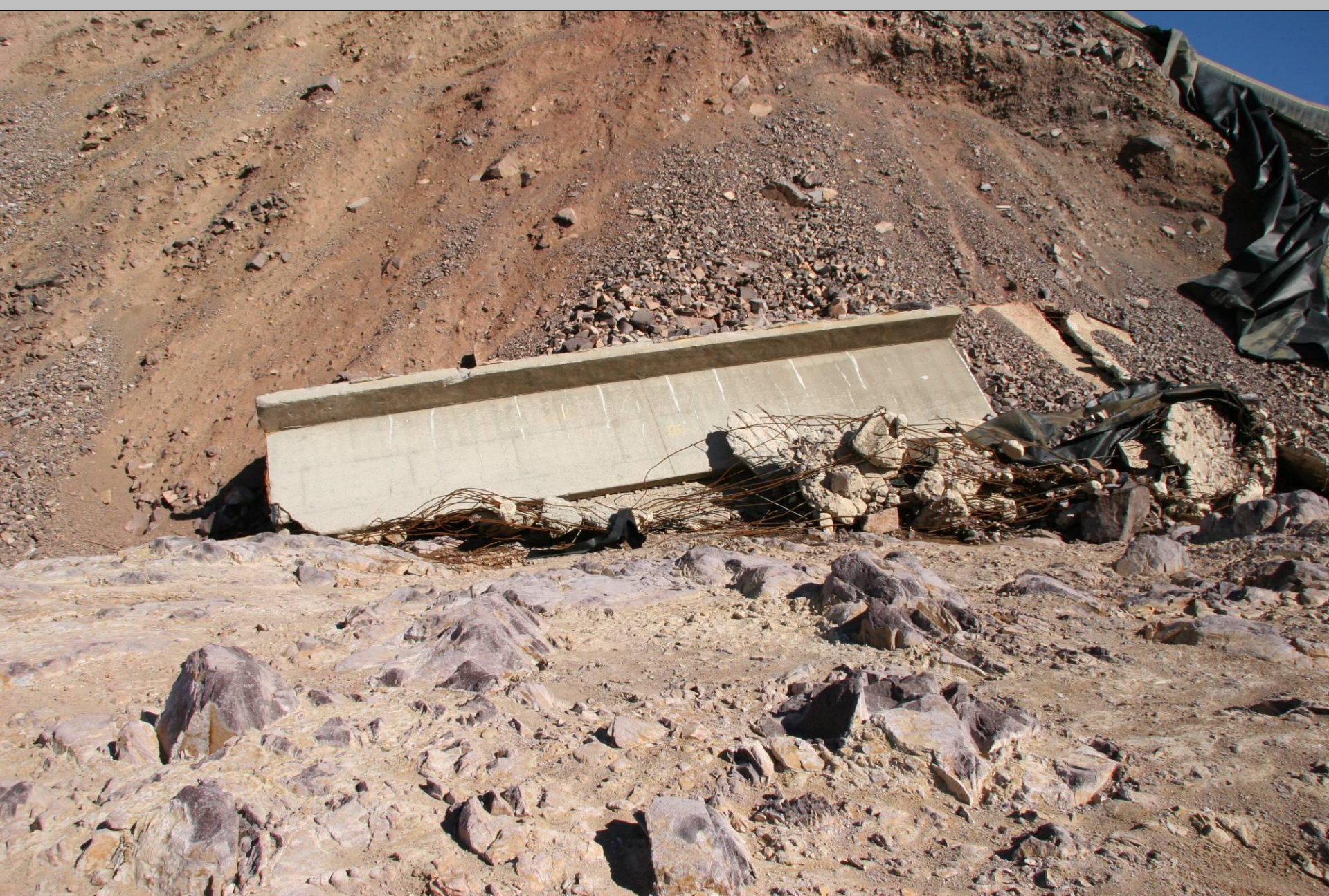
Toppled wall panel at north end of breach. The stem was 10 feet high.
