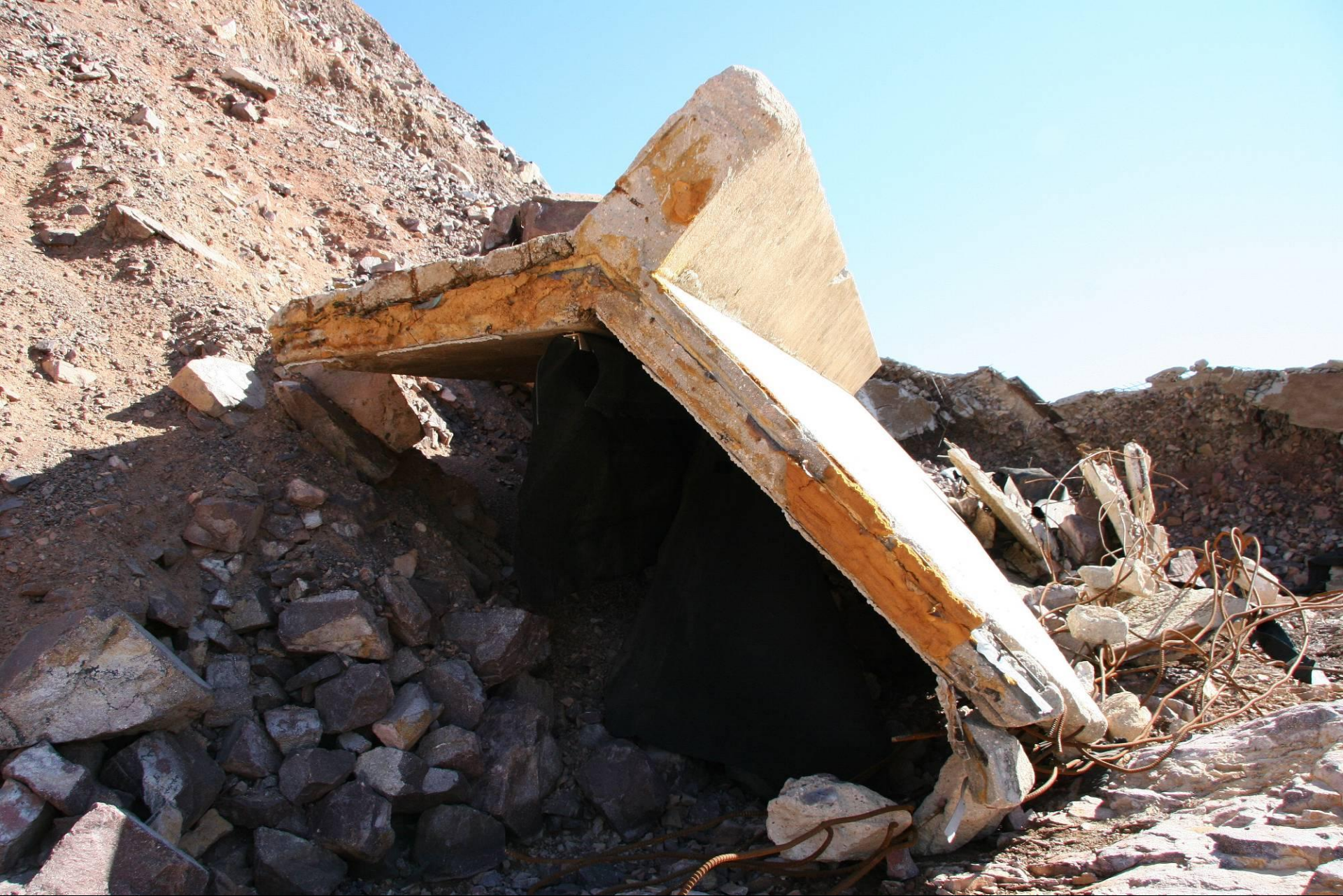
Wall panels toppled over after extensive undercutting, initiating the catastrophic failure sequence.
