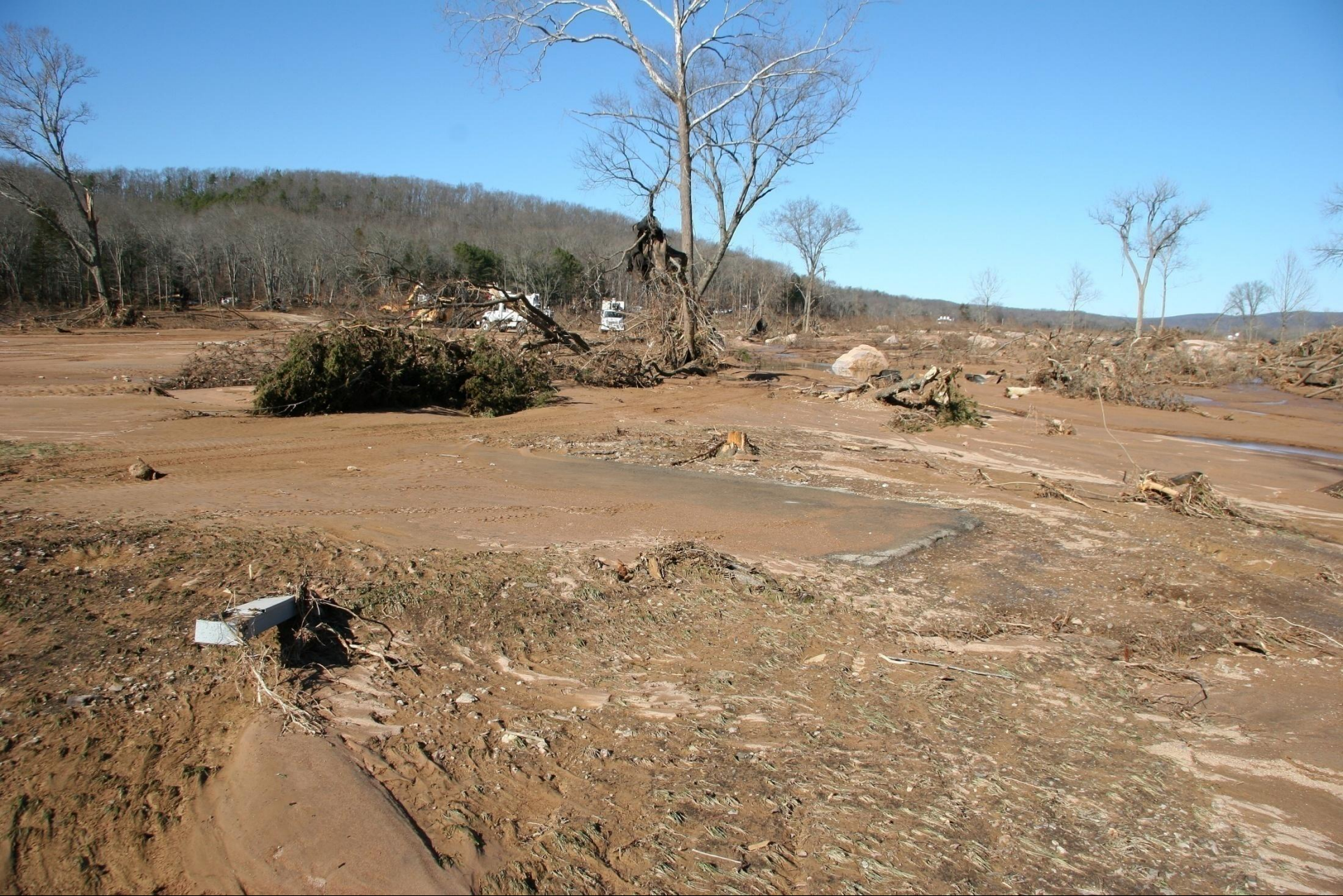
Deposition of boulders, mud, and trees in the campground at Johnson's Shut-ins State Park.
