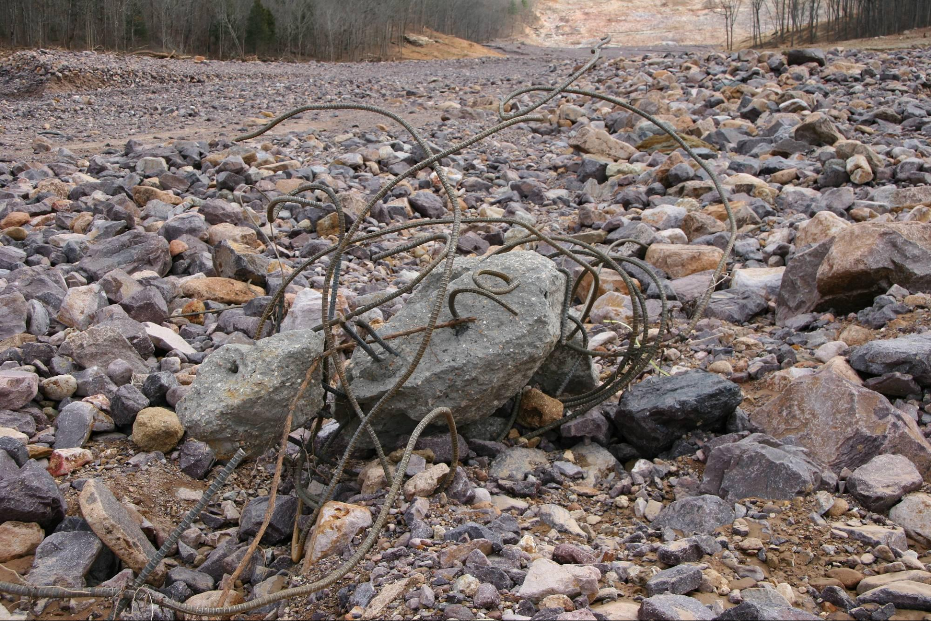
Concrete and rebar from the dike littered the scour channel.
