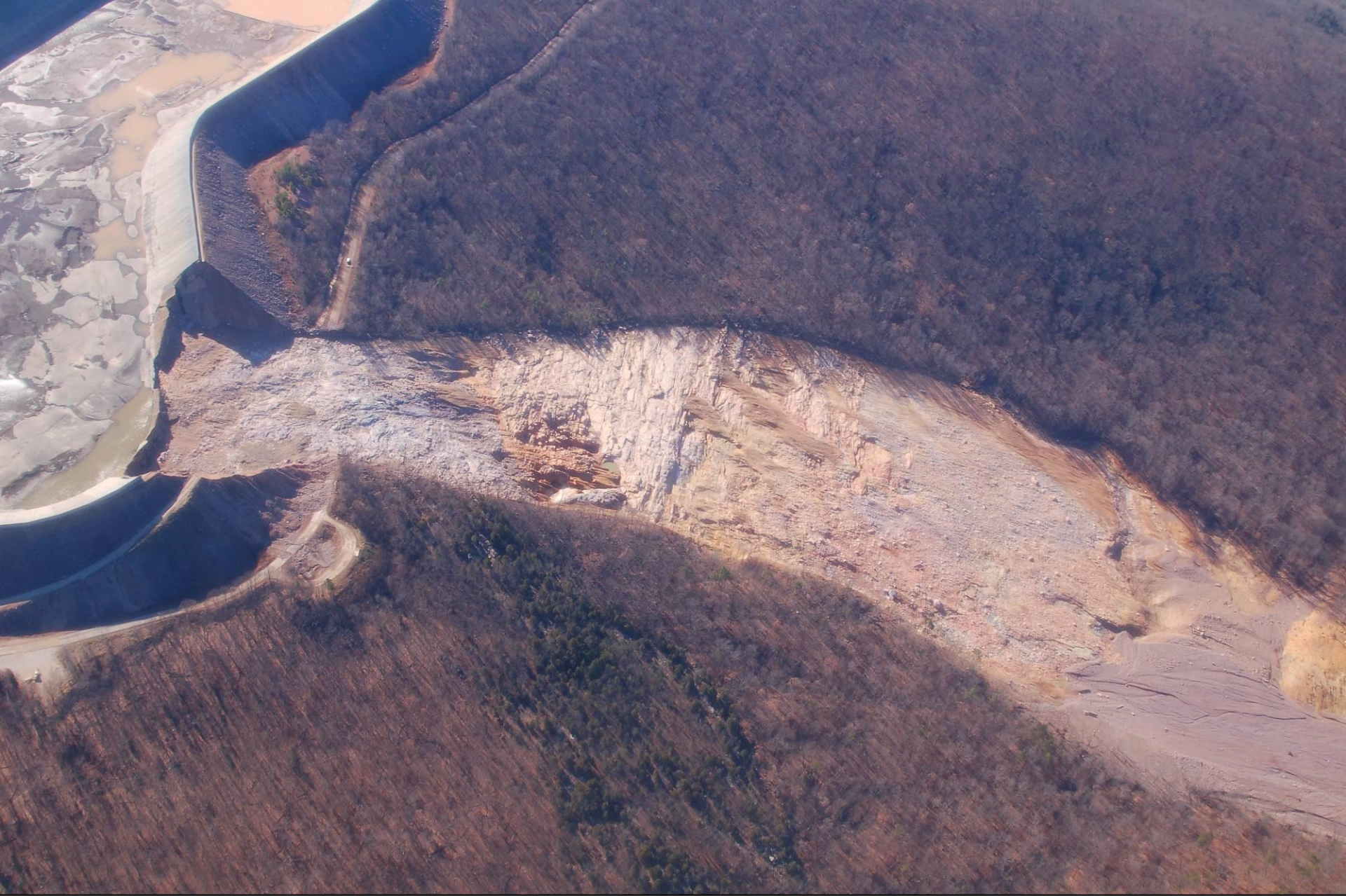
The flow path down the slope of Proffit Mountain was stripped down to the underlying bedrock (photo by Jeff Spooner (USGS)).
