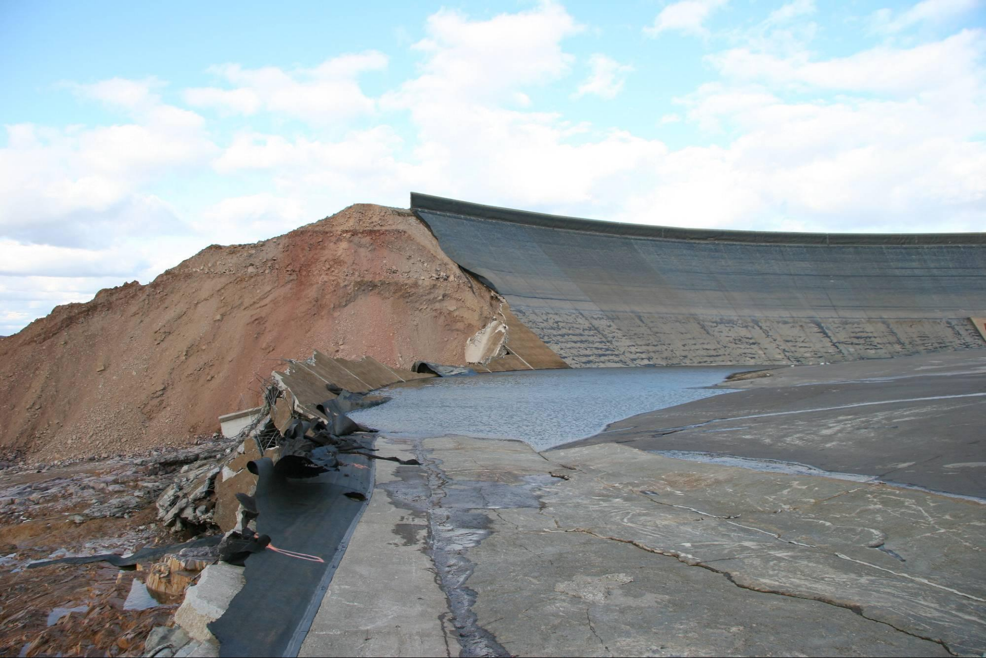
A small lip of material armored by portions of the concrete liner remained in a few locations at the breach site.
