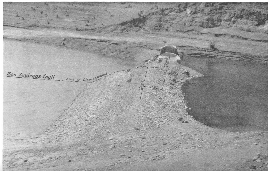
Fig. 2. View along the axis of the old dam in the San Andreas Valley (the same as fig. 1), showing the offset of about seven feet caused by the fault movement of April 18, 1906.
