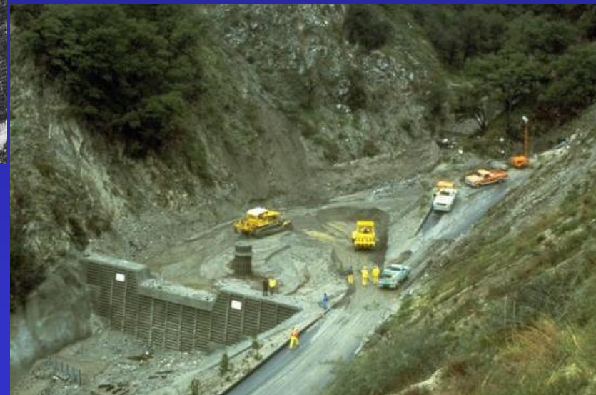
Crews mucking out a small debris basin in Los Angeles County. Note perforated riser intake tower.
