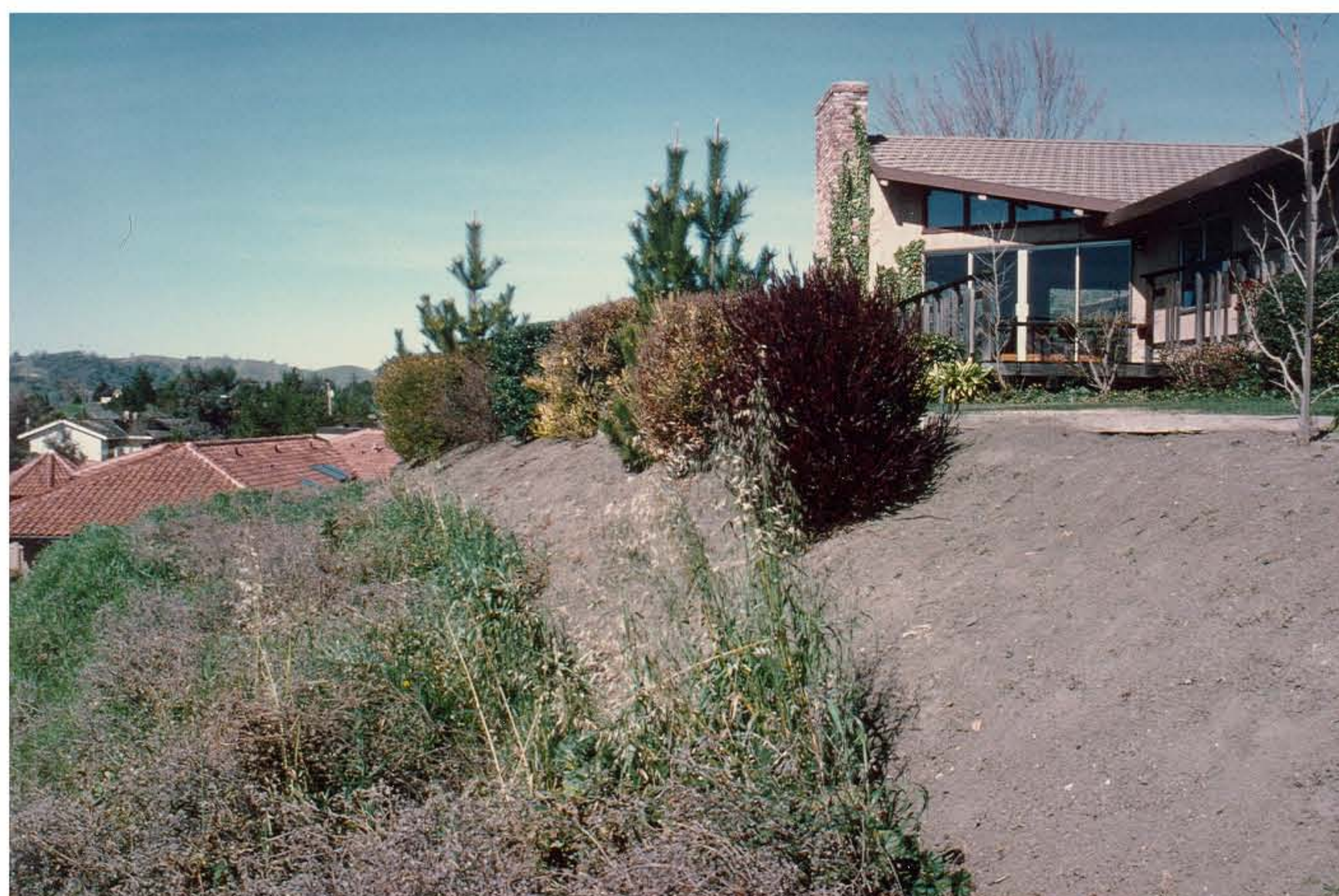
Figure 3. A: Overview of the Easton home, situated in the community of Diablo, Contra Costa County, California. B: Ground view at brow of the fill slope behind the Easton home. It was this slope that had supposedly settled. The California Supreme Court found the realtor guilty on the premise that they should have made themselves aware of the settling problem by simply viewing the slope in combination with the knowledge that the home was built upon fill. The court did not accept any expert testimony from geotechnical professionals regarding the veracity of such a premise.
