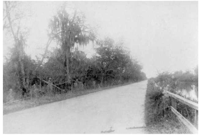
Fig. 10. Photo taken in 1890 looking north along “shell road” that ran along west side of New Basin Canal, seen at extreme right. Note modest height of original embankment, no more than 1.5 m above adjacent cypress swamp at left. Canal levees were heightened after hurricanes in 1915 and 1947. (Image from University of New Orleans special collections)
