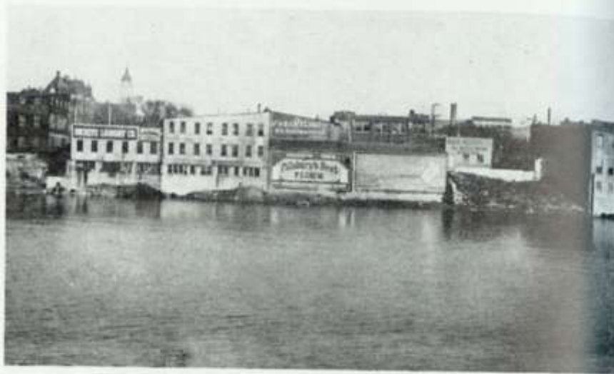
River channel at Hamilton before improvement.
