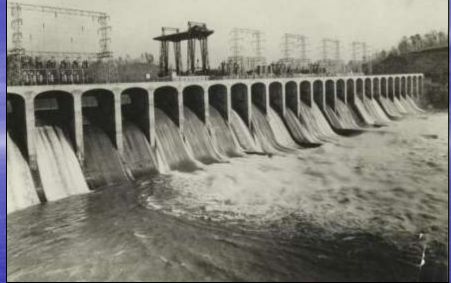
Wilson Dam was built between 1918-25, but the hydroelectric generation plants were privately operated.
