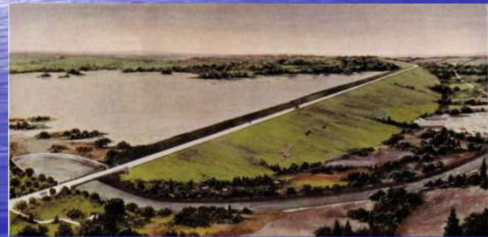
Color concept renderings prepared by Morgan in 1914. The central service spillway was un-gated, while the auxiliary spillway sill was situated 15 feet below crest.
