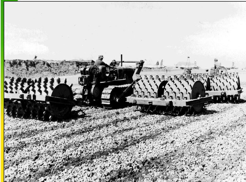
Tandem hammerhead Sheepsfoot rollers (above right) being used to compact runway gravel subgrade on Iwo Jima in June 1945
