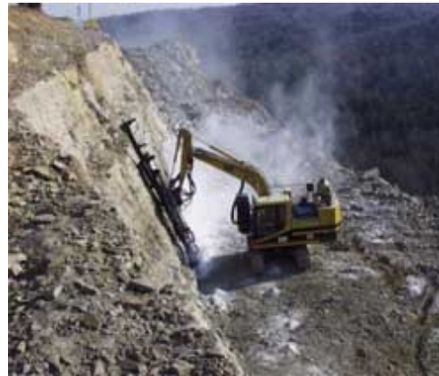
Drilling presplit holes
