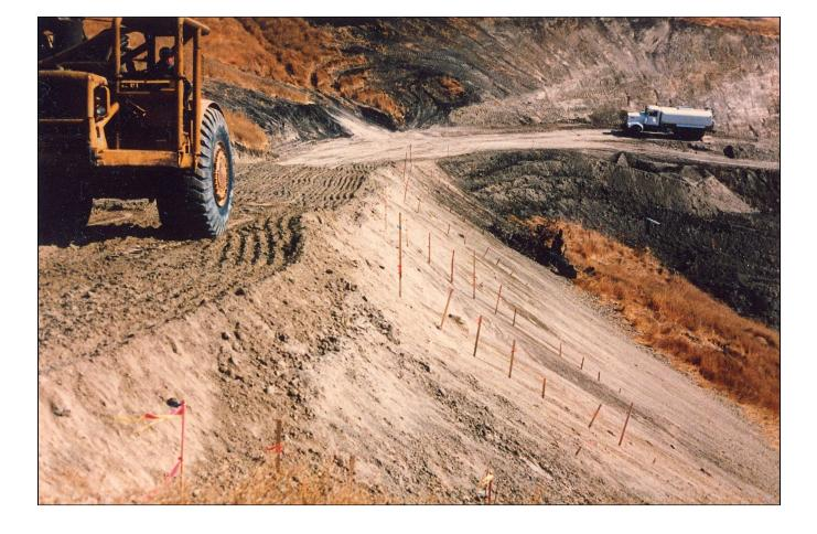
Construction of 45 degree sidehill embankment for a road in steep terrain. Both false and full-depth geotextile mats were incorporated into the embankment, spaced every 12 inches.
