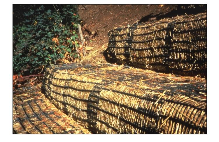
Geogrid-wrapped hay bales can be used as temporary facing elements for mechanically-stabilized embankments. These materials do not corrode, so are perceived to be more "environmentally friendly."
