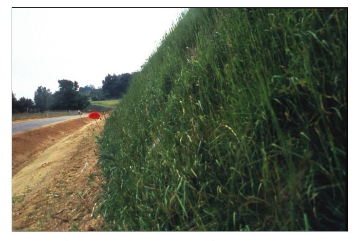
Fiber reinforced soil wall after grass cover has germinated. The fiberglass roving is an effective tackifier, promoting seed adhesion and root penetration
