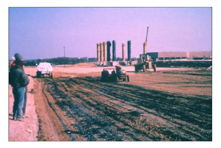
Geofibers can be mixed with subgrade soils, as shown above. Their inclusion raises the maximum density about 5% and reduces the optimum moisture content of the compacted soil mixture about 5% as well.
