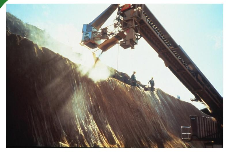
The sand and fiber mixture can be sprayed onto a problem slope like shotcrete, creating a free-draining gravity retention structure. The roving is typically applied at a nominal rate of 20 m/sec.
