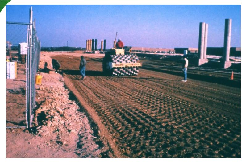
Geofibers are compacted into the soil using kneading compaction for cohesive soils and vibratory rollers for granular mixtures.
