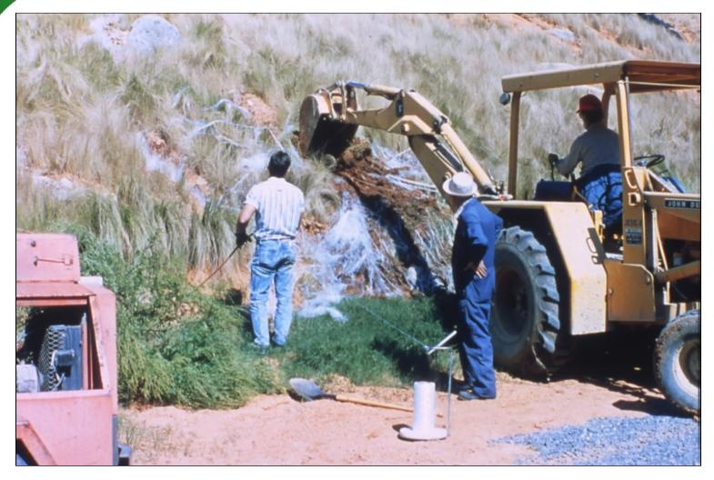
Backhoe cutting inspection trench into the treated slope a year or so later, after vegetation had taken hold. Revegetation is increasingly valued for aesthetic reasons.
