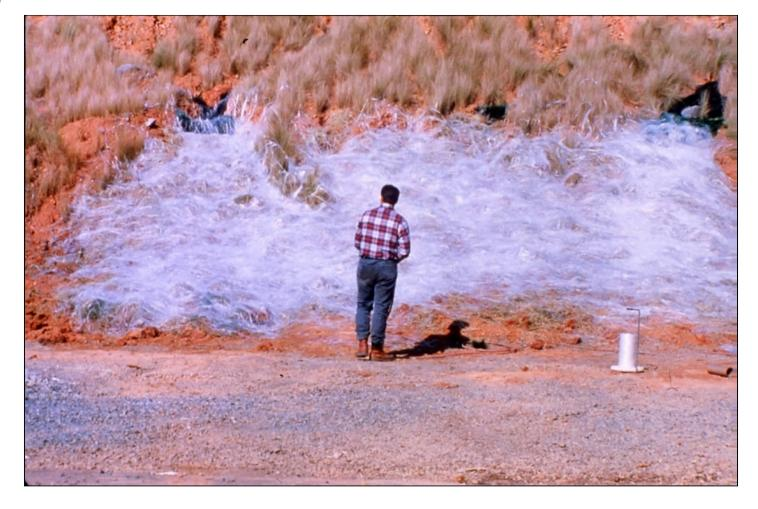
Test block using Geofiber-reinforced soil mixture sprayed onto the eroded cut slope, infilling the erosion gullies
