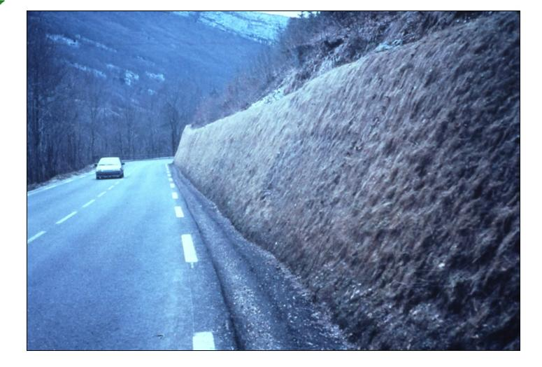
Texsol fiber reinforced soil retaining wall shortly after construction, along existing mountain highway in Europe.
