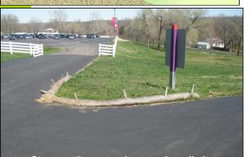
Straw wattles are an inexpensive, albeit temporary, means of deflecting sheet flow from paved surfaces
