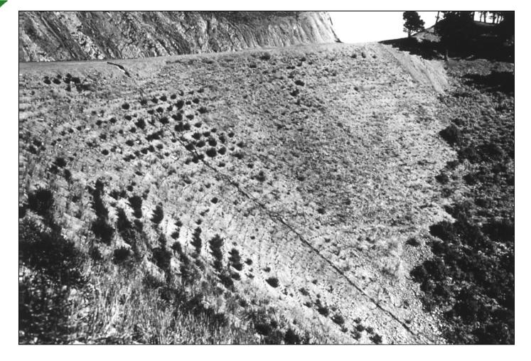
Growth of willow wattles planted on Grizzly Peak fill slope during summer of 1935. The wattles were not irrigated during 7 months of dry weather, so losses were significant.
