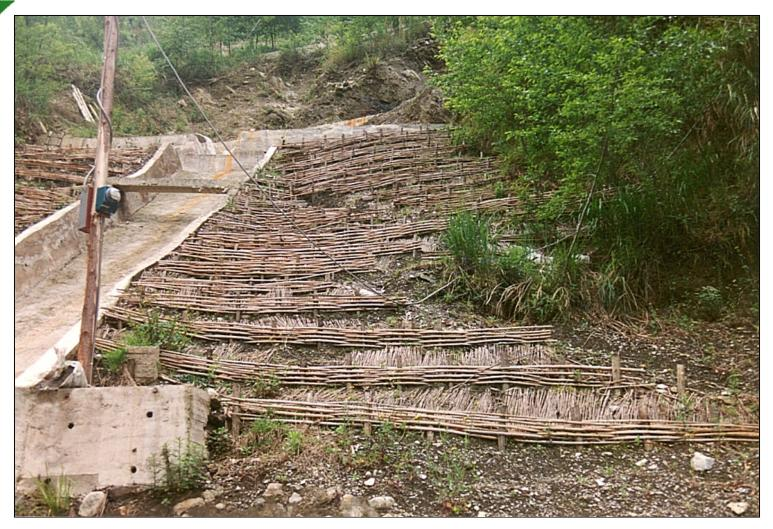
Bamboo fascines are used extensively to protect cut slopes in Asia, such as this example in Taiwan. In Europe fascines are usually made of creek willow chutes.
