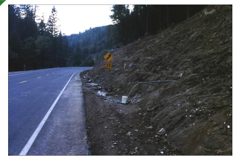
Discharge from hydrauger drains can easily be measured using a 5 gallon bucket, as shown here. Discharge as great as 1 million gpd have been documented over the years.
