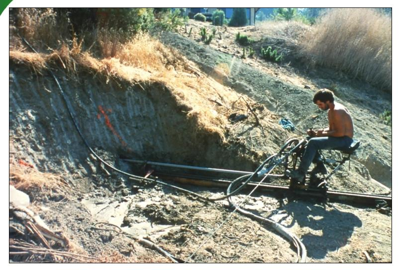
Some home-built hydraugers can be broken down into lightweight components, which can be re-assembled in remote locations, like that shown here, which is powered by hydraulics from a compressor located at the crest of the slope.
