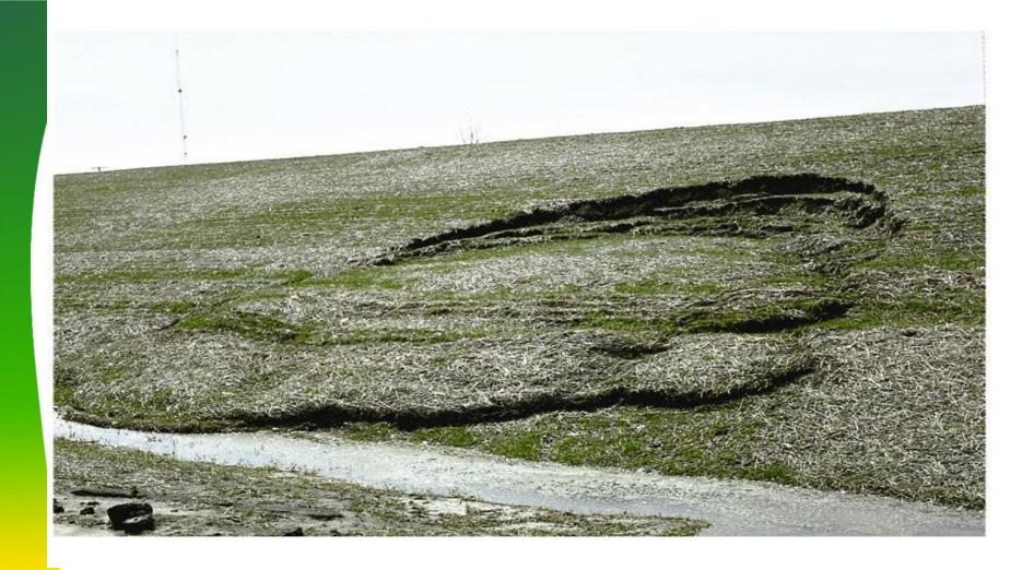
Rotational slump-flow of a newly graded embankment along the westbound onramp of Interstate 44 in Rolla, MO. This slump was triggered by concentrated seepage along a single joint cluster, where they intersected a pervious bed
