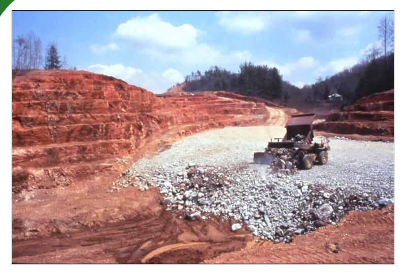
Blanket drains are used beneath embankments in areas where clean rock is readily available and thorough underdrainage is desired.
