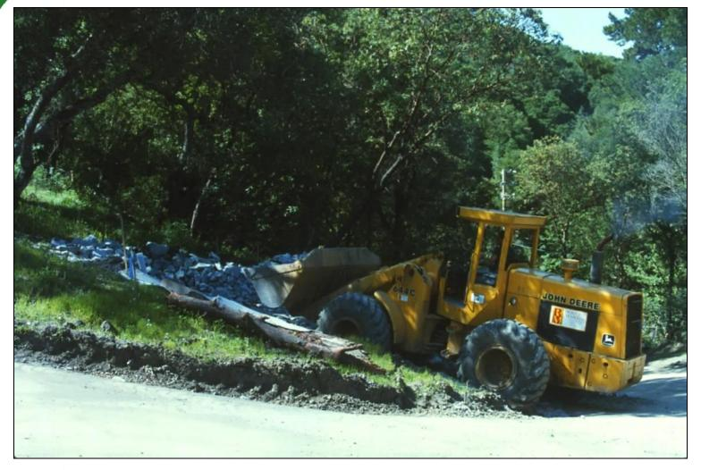
Rubber tired skip loader placing 12" x 18" armor rock over a geotextile filter cloth as part of a small slope repair
