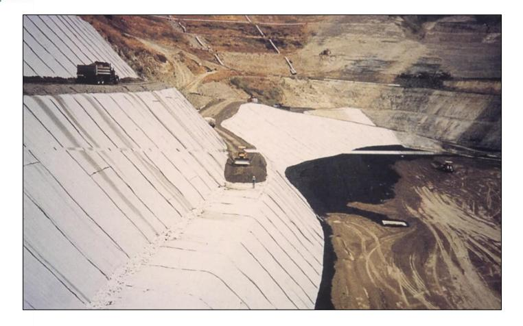
Gravel bench drains being spread over geotextile filter fabric in a sanitary landfill. Impervious membranes are often placed beneath these drains to trap and convey seepage or leachates to a controlled point of discharge
