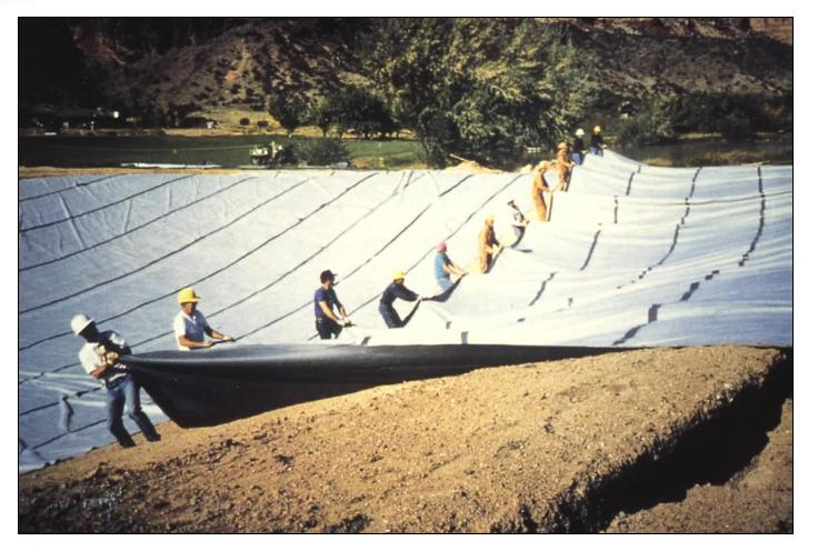
A plethora of geotextile filter fabrics are available for employment beneath fills for structures, highways or landfills. They must be properly lapped and keyed into the subgrade
