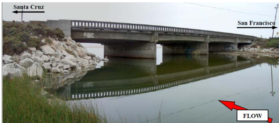
Figure 1 Highway No.1 Waddell Creek Bridge
