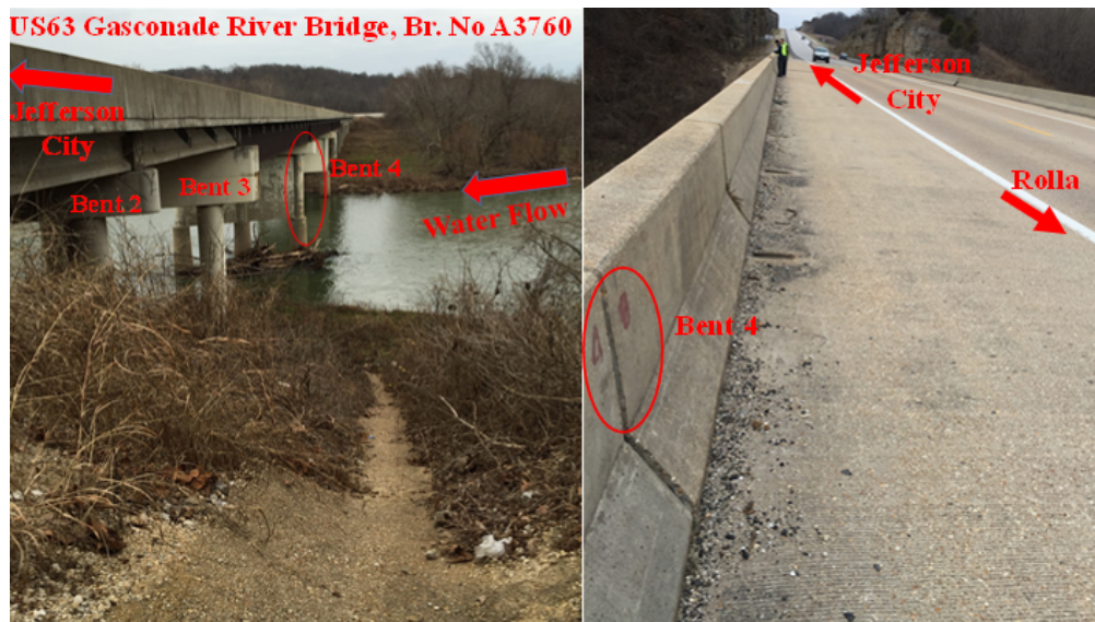
Figure 1 The US63 HWY Gasconade River Bridge
