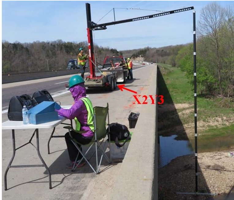
(a) Test Crane Located at Y2X2
