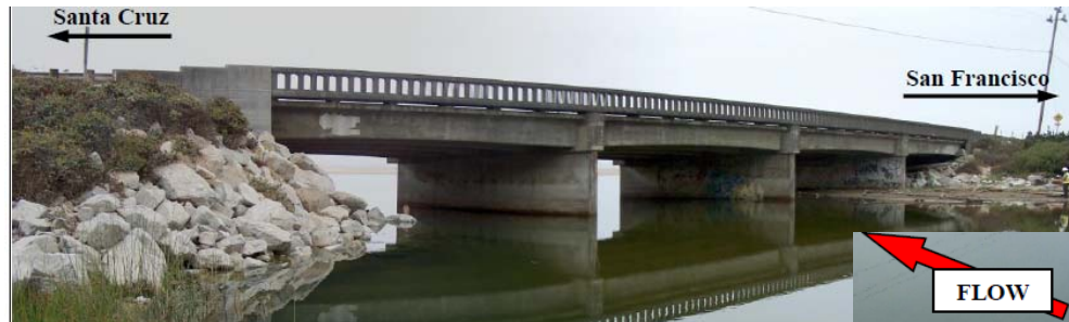
Figure 2.5. State Hwy1 Bridge over the Waddell Creek.
