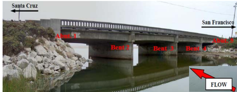
Figure 5.12. State Highway 1 Bridge over Waddell Creek, CA.
