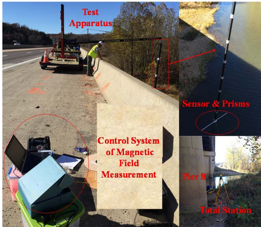
(b) Overview of the Entire Measurement System
