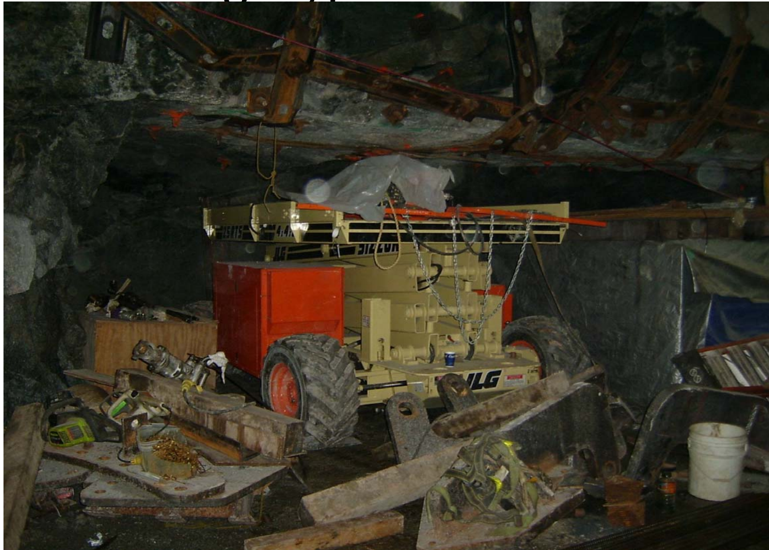
Housing new main bearing and man-lift
