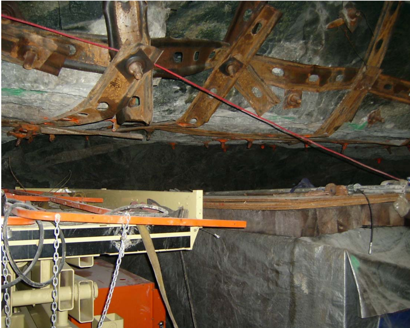
Supporting roof bypass cavern
