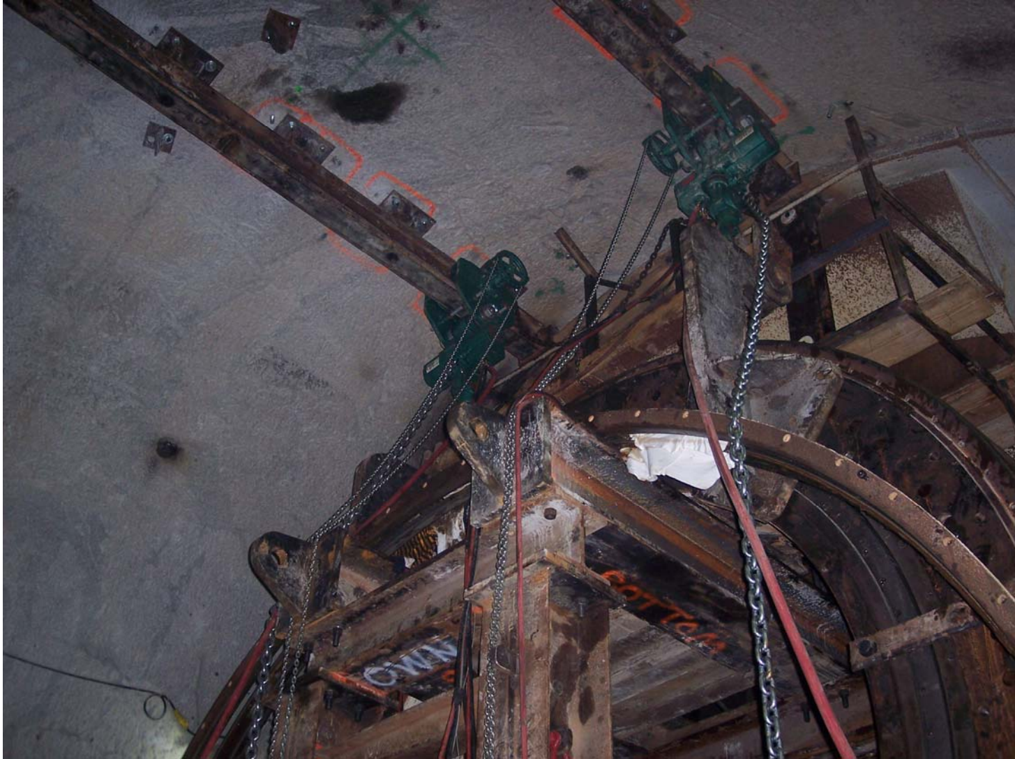
50 ton monorail system to lift and move main bearing
