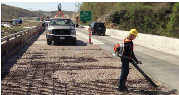
Figure 10: Bridge deck scanning after hydrodemolition.
