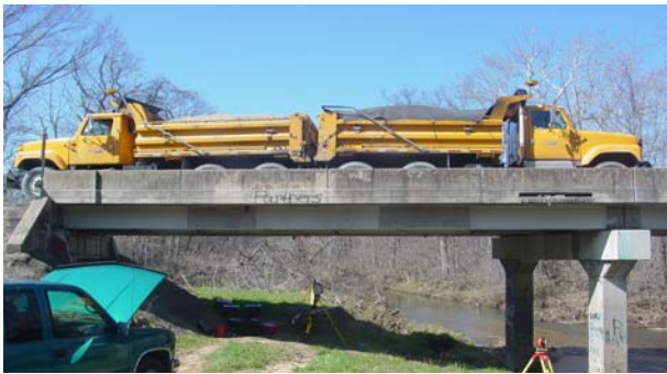
Figure 2: Bridge span loaded with gravel filled trucks.
