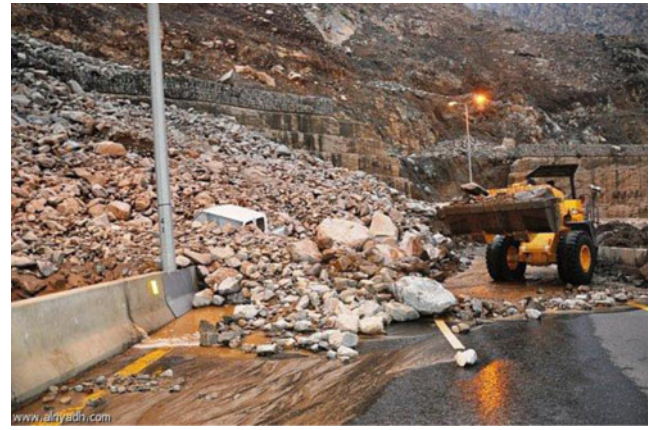
Fig. 6 Removing the debris from the road along site 1
