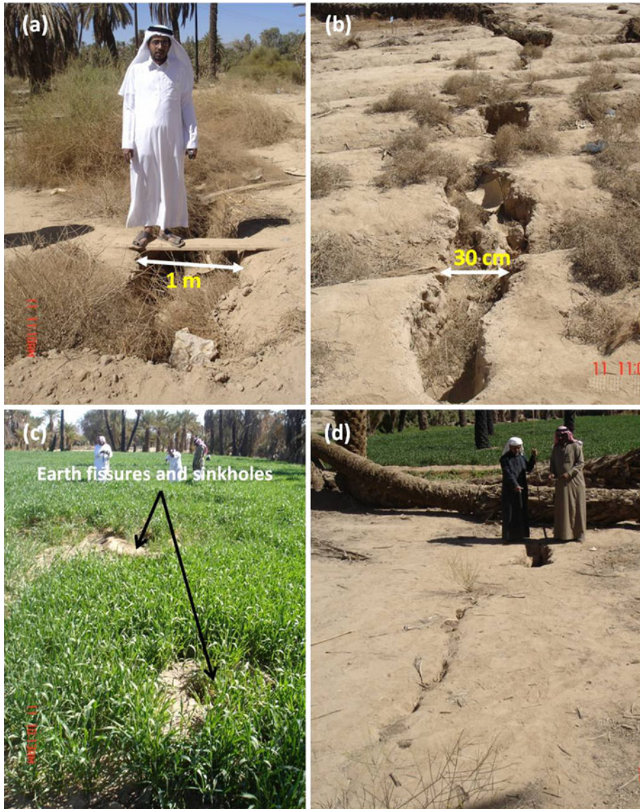
Fig. 2 Fissuring associated with subsidence due to groundwater withdrawal in Najran ( a and b ) in an uninhabited area and ( c and d ) in agricultural fields
