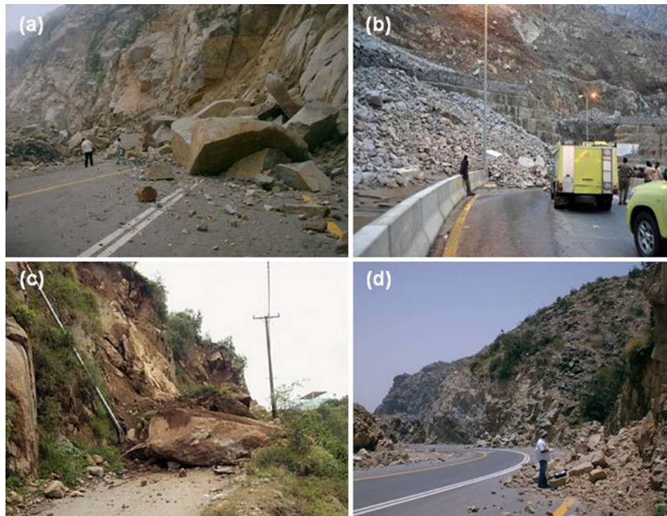
Fig. 6 a Rock falls along the Al-Hada highway; b debris flow along Al-Hada Highway; and c slope failure in Jazan; d slope failure in Taeif
