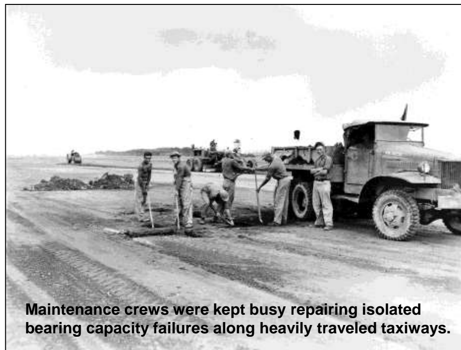
By the war's end in August 1945, Yonton Field on Okinawa was being constructed with a well-graded mix of crushed coral 30 inches thick!
