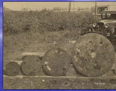
In the late 1920s foundation engineering basically revolved around the application of plate load tests in hand excavated test pits. The sizes and shapes of the plates were varied according to the need, as was the depth of the pit
