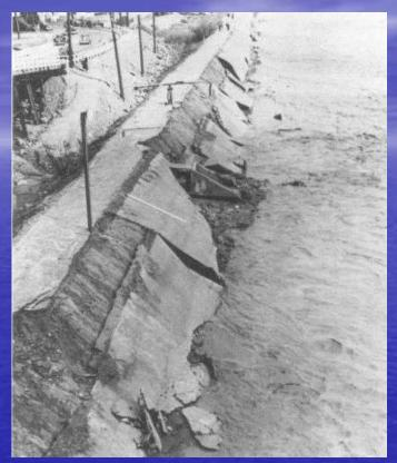
Damage like that shown above along the channelized Los Angeles River in the March 1938 flood spurred the Federal Flood Control Acts of 1936, 1941 and 1944, which placed the U.S. Corps of Engineers into a prominent role to help provide flood control nationwide, on a 65/35 shared cost basis with local agencies.
