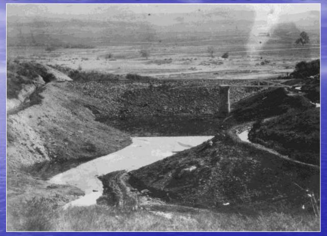
Buena Vista Reservoir was constructed in 1868-69 using an earthfill embankment with riprap face, built to a crest elevation of 378 feet. It was located near what is now the southeastern tip of Elysian Park, in Los Angeles. It was owned by the Los Angeles Water Company as their first storage facility. This area is now part of Buena Vista Park, just off the Pasadena Freeway.
