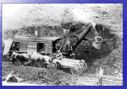
Note the old Buffalo-Springfield steam roller compacting the dam's embankment, in left background. Below Left: Marion shovel loading a hopper dumping wagon at the San Pablo Dam site of the East Bay Water Company in 1920, near Richmond, California. At 220 ft high with a volume of 2.2 million yds<sup>3</sup>, it was the highest and largest earth dam in the world when completed in 1922.
