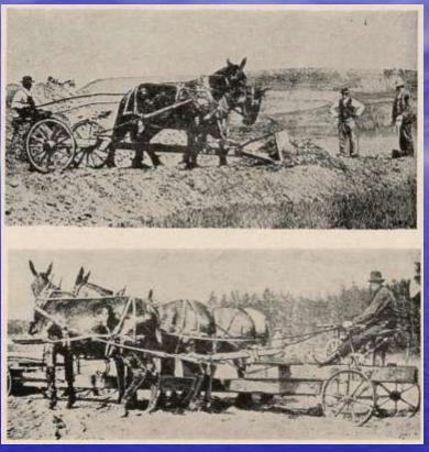
The Bulldozer was developed in the late 19<sup>th</sup> Century to grade railroad lines. Two bulls or horses (upper right), or up to 4 mules (lower right), could be employed to pull a wheeled caisson attached to a stiff arm connected to a flat iron blade, which extended out in front of the animals, as shown above. The advertisement at left is from the Western Wheeled Scraper Co., in 1917.
