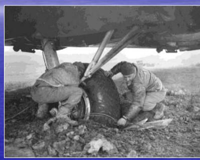
During World War II, the Corps of Engineers noted an increasing problem with pavement distress near the edges of heavily traveled taxiways. The weak link appeared to be subgrade preparation (images from 401st Bomb Group at Deenethorpe, UK)
