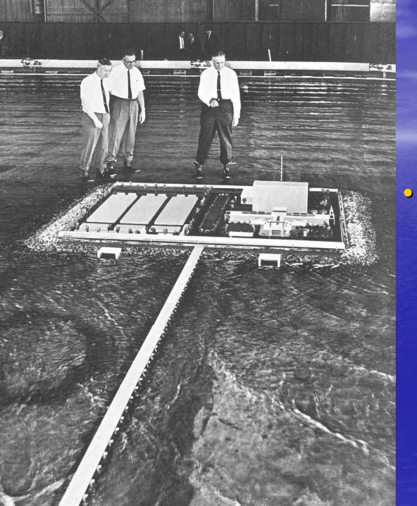
Bolsa Nuclear Power & Desal Plant One of the most challenging projects of the 1960s was MWD's proposed Bolsa nuclear power and desalination plant, which would have been situated offshore
