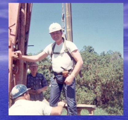
Around 1960 several southland geologists began using large diameter bucket auger excavations to assess complex geologic conditions. This became the preferred method of site exploration over the following decade.
