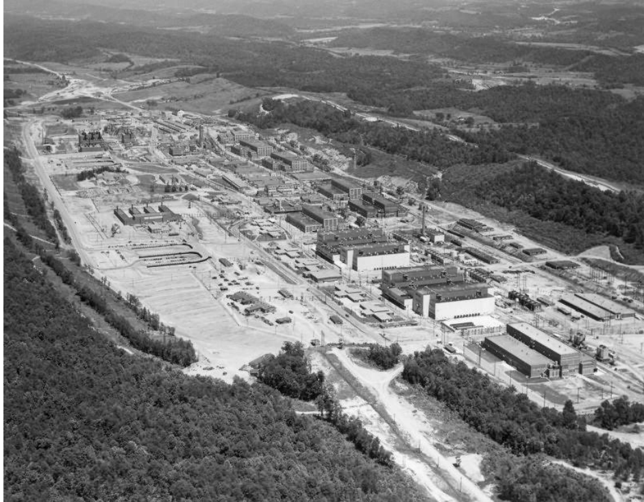
The massive Y-12 plant at Oak Ridge, Tennessee was designed and built in record time by the legendary Boston engineering firm Stone & Webster.
