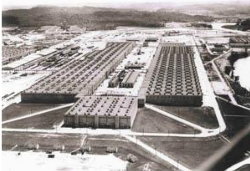
K-25 Plant at Oak Ridge. This U-shaped facility was 2,500 feet long on each side, 450 feet wide, and 60 feet high, occupying 44 acres. Here uranium hexafluoride ( \text{UF}_6 ) was forced through 3,000 stages in a continuous cascade, to slowly filter out the lighter U-235 atoms.
