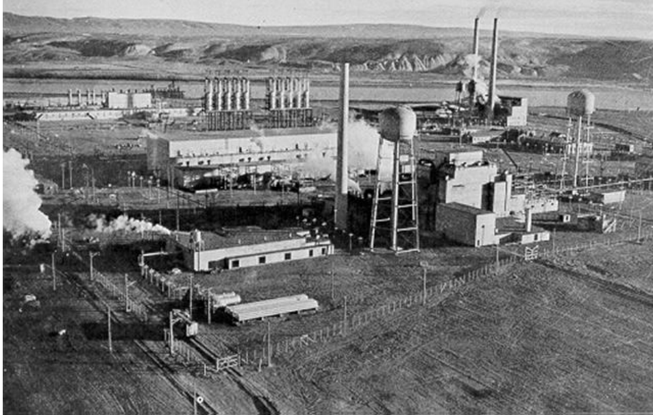
The B Reactor complex was the first constructed at Hanford, Washington, coming on-line in September 1944. Plutonium production fell to near zero on several occasions, and Enrico Fermi and his team had to troubleshoot the problems and develop workable protocols to maintain output during the war.
