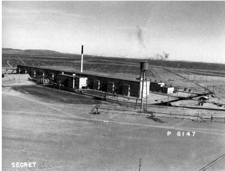
The T Plant at Hanford was completed in December 1944 as the world's first large-scale plutonium separation facility. Only about one atom in 4,000 was converted to plutonium in the three Hanford production reactors, so these atoms had to be separated from the remaining U238 and other fission products that had been created.
