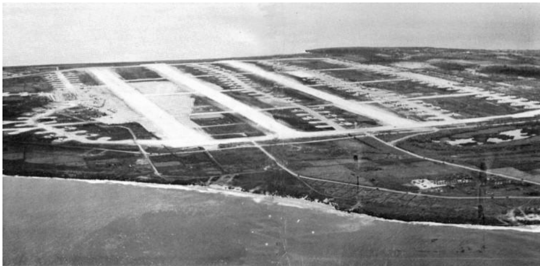
The North Field complex on Tinian Island in the Mariannas. Eventually equipped with four 8,500 foot runways and 265 hardstands, North Field was the largest airdrome constructed during World War II. The atomic missions were flown from this base, with the 509 th Group occupying the area at extreme left in this image.
