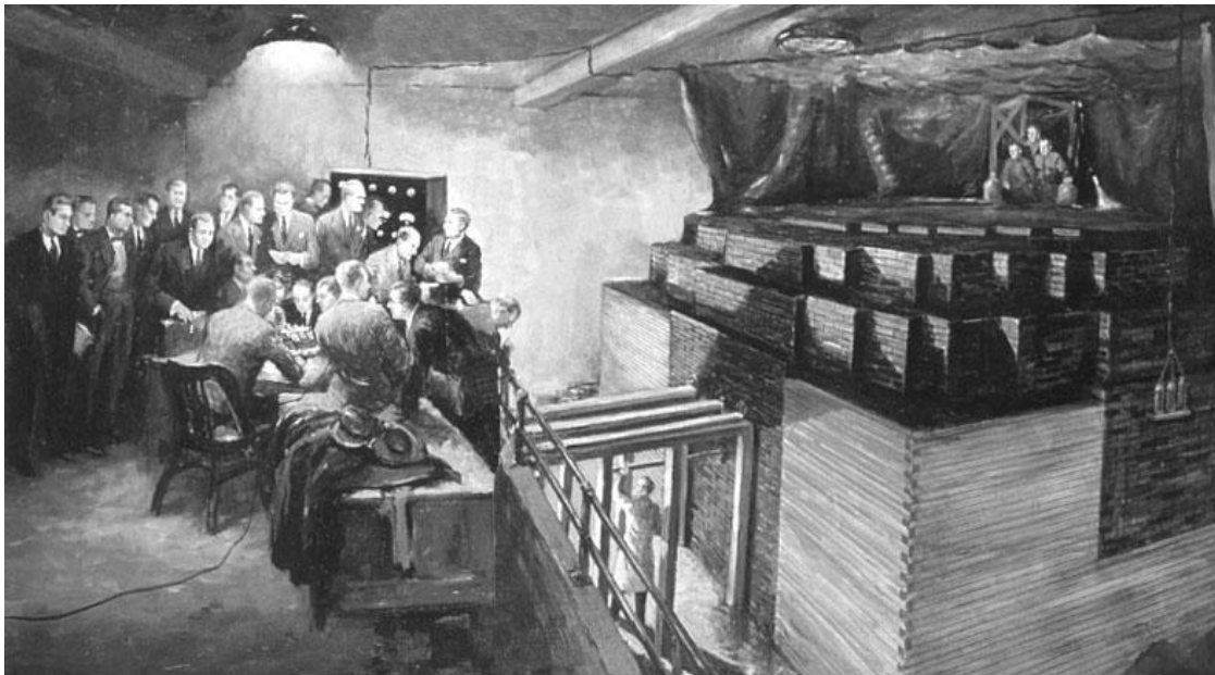
The world's first successful nuclear reactor was constructed on a squash court beneath the bleachers of Stagg Field at the University of Chicago. It incorporated 40,000 blocks of pure graphite, weighing 500 tons, provided by Union Carbide. The first successful chain reaction was recorded on December 2, 1942, six months after the German reactor in Leipzig caught fire and was destroyed.
