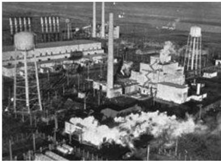
Hanford B Plant separation and enrichment facility, as seen in 1945.
