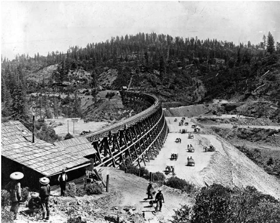
Judah's route ascending the crest of the Sierras at Donner Summit depended on maintaining an increasing grade at every point along the line. This was achieved in large measure by backfilling timber trestles with fill from adjacent cuts using small dump carts, as seen here at Secretown.
