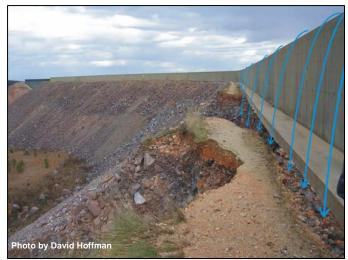
Fig 9. – This photograph shows arrows representing the overflow nappe once it extended beyond the 3 foot wide wall footing and directly onto the underlying rockfill. The rate of scour and erosion increased dramatically once this occurred.
