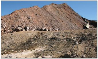
Fig. 21. – Residual soils, including tree roots and other organic matter, were observed left in place beneath the failed portion of the upper reservoir embankment.
