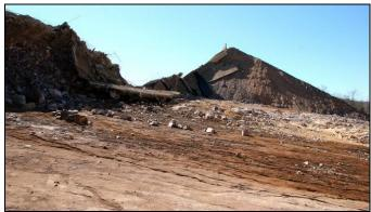
*Fig.* 18. – *The remnant lip as seen at the failure site.*
