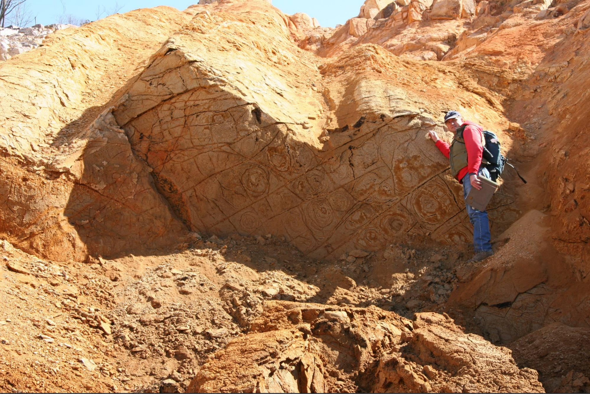
This diabase dike (or sill) on the upper slopes of Proffit Mountain weathered to a weak soil-like material, yet retained the rock's original fabric and fracture pattern.
