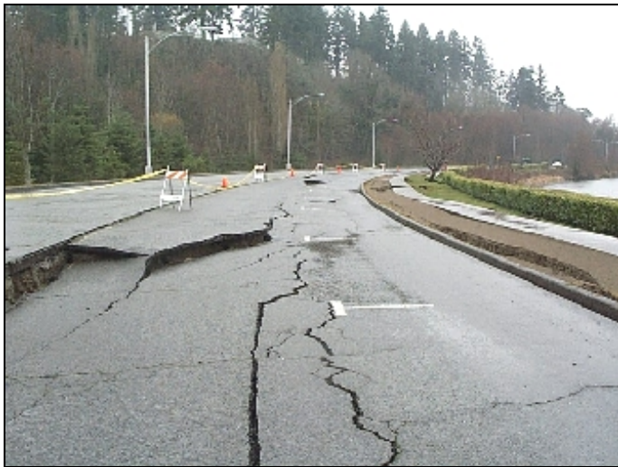
Fig. 23 – Example photo documenting site damage, imaged along North Deschutes Parkway showing a lateral spread toward Capitol Lake, which is to the right of the photograph. All photos were georeferenced and dated (from Bray, et al, 2001).
