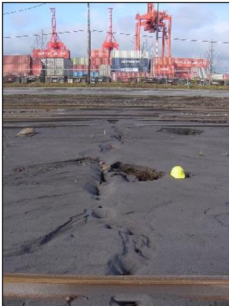
Fig. 20. Sand ejected from a ground fissure crossing railroad tracks at the Port of Seattle. The opening was found to run through the road into the port facilities seen in the background. All ground photos were georeferenced using GPS receivers (N47.58487° W122.33980°), (from Bray, et al, 2001).
