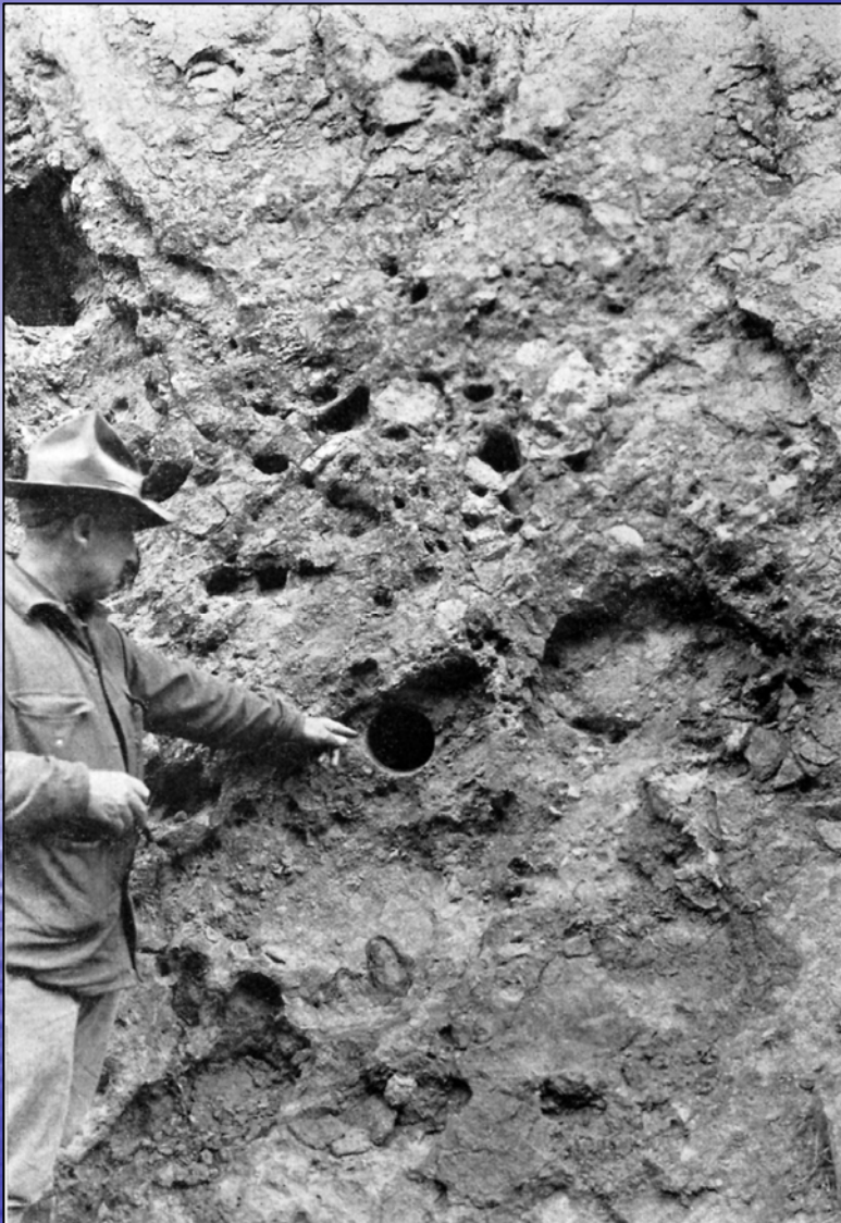
6-inch cores were extracted from the abutments for unconfined compression tests
