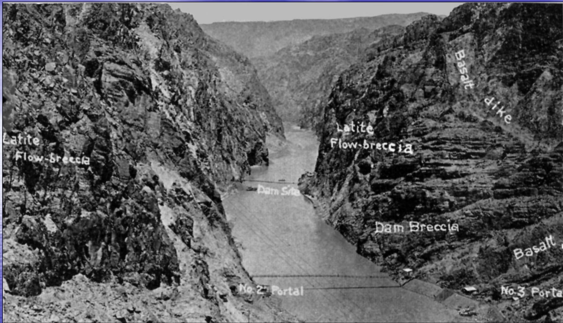
View of dam site looking upstream, annotated with geology. Note basalt dike at right, on Arizona abutment. These dikes perturbed both abutments.
