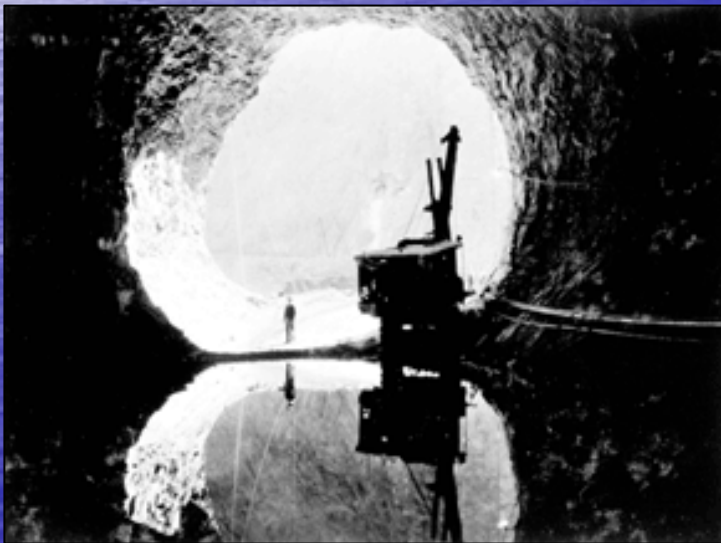
Finished 56 foot diameter bore
