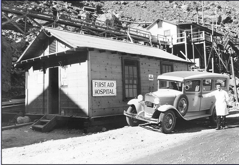
Emergency room built on job site
