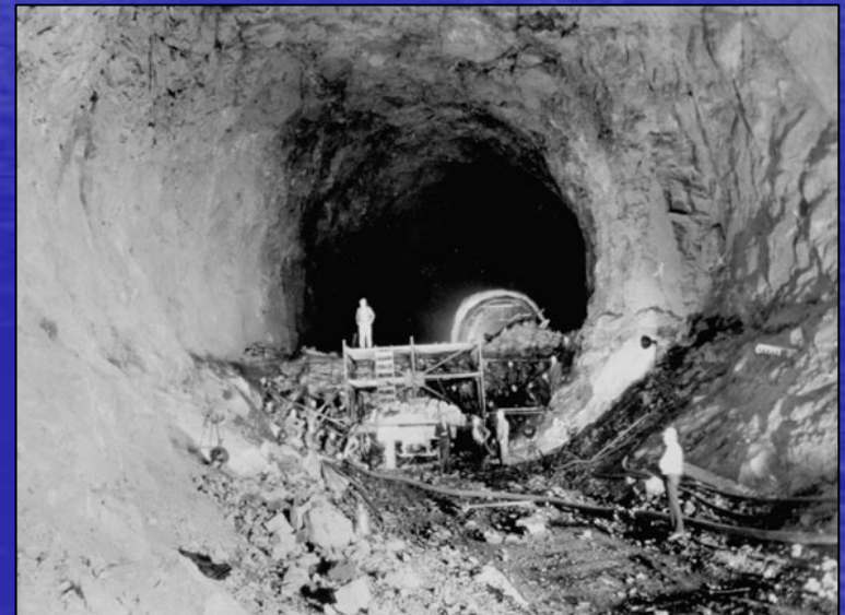
Ready for lining
