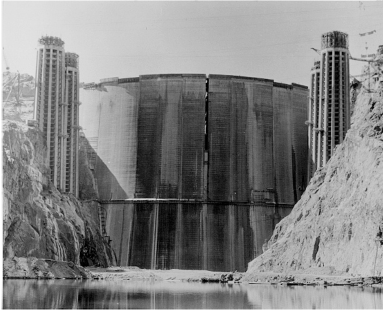
FIG. 28. 8-foot-wide “cooling slot” running vertically through the dam’s axis afforded temporary access to the dam’s cooling pipes until the concrete’s heat of hydration was brought down to acceptable levels. This was grouted with a standard mix in 10 ft increments as the dam rose upward. (USBR)
