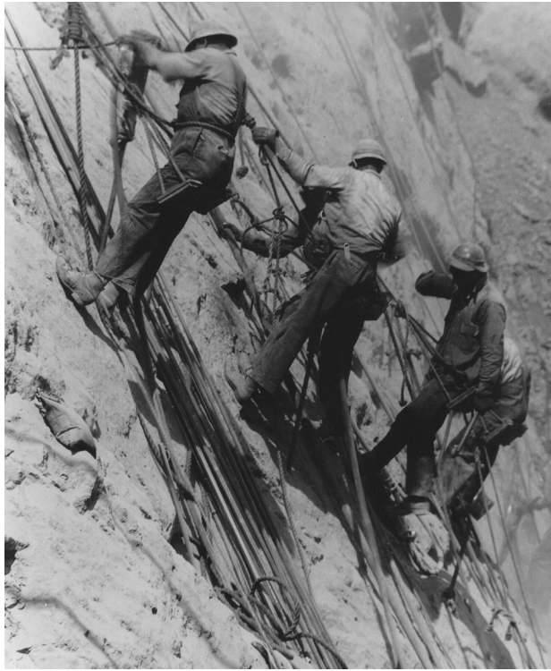
FIG. 16. High Scalers in Bosun’s Chairs operating jackhammers to drill holes for production blasting. This was hot, dirty, rough work, without any chance for rest. On the very steep slopes, like that shown here, scalers would have to stop and help one another ‘set up’ their ‘jacklegs’ on a hole and drill it a sufficient distance so that a man could safely control it (USBR).
