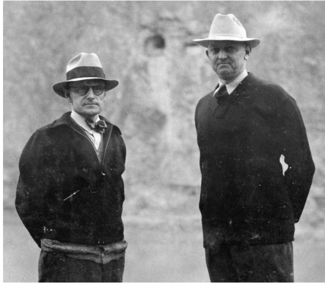
FIG. 1. Civil engineers Walker R. Young (left) and Frank T. Crowe (right). Young was the senior onsite representative (Construction Engineer) for the Bureau of Reclamation while Crowe was the General Superintendent for Six Companies (USBR photo). Everyone expected Young to succeed Elwood Mead as the next Commissioner of Reclamation, but his subordinate John C. Page was given the position because he was a Democrat. Crowe went on to manage construction of Parker and Shasta Dams before dying of a heart attack at age 63 in February 1946. Young went on to head up the Central Valley Project in California, returning to Reclamation headquarters in 1945, where he served as Assistant Chief and then Chief Engineer until retiring in 1948. He lived to be 97, passing away in 1982.
