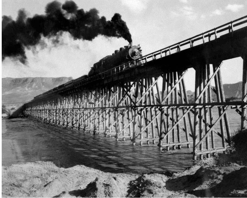
FIG. 30. Six Companies Inc. railroad train hauling aggregate from the terrace gravel deposits in Arizona across the Colorado River on a temporary timber trestle. This trestle survived all of the high flows until it was dismantled in the fall of 1934 (Six Companies Collection, USBR-LCR).
