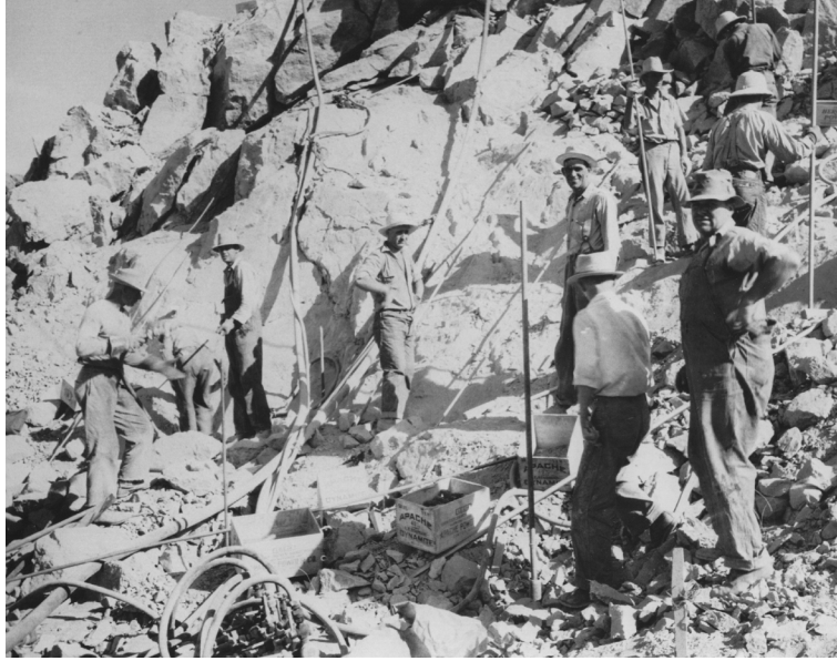
FIG. 17. A group of ‘powder monkeys’ loading drill holes with dynamite, stemming, and blasting caps, photographed on August 15, 1932. Note the thin steel tamping bars, which were typically 10 ft long. These were used to tamp the sticks of dynamite and pack the stemming in the upper part of the holes, to force the blast energy into the rock mass (Bechtel Collection, USBR).
