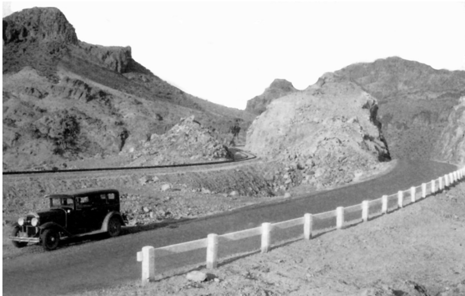
FIG. 3. Upper: The R.G. LeTourneau Co. lost close to $100,000 while grading the government highway between Boulder City and the dam staging area because they encountered resistant volcanic strata that proved much more troublesome than anything they had previously dealt with in California. The lower image shows the completed highway (costing $330,000) with the U.S. Construction Railroad in the background (costing $1 million). (USBR)
