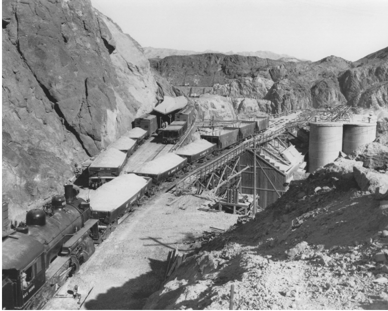
FIG. 33. Classified aggregate being delivered to hoppers at the High-Level Mixing Plant by the Six Companies Inc. Railroad at an elevation of 1403 ft. The aggregate came from the classification plant in Hemenway Wash (USBR-LCR).
