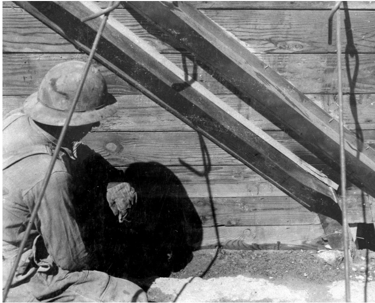
FIG. 34. Six Companies worker wearing one of the mass-produced hard hats they issued free-of-charge to their workers, encouraging them to wear them wherever loose materials might fall upon them. They purchased five different kinds of hard hats, from different suppliers/manufacturers (USBR).
