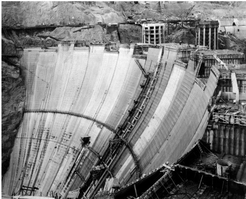
FIG. 12. Hoover Dam nearing completion, as seen along the downstream face, around New Years 1935. Note the vertical slot at midstream, which was not filled until after cooling water circulation was completed in mid-March 1935 (USBR).
