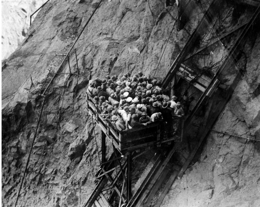
FIG. 29. 80 men being taken down the 10 by 12 ft skiff on the Nevada Abutment, heading to work on the 4 PM to Midnight swing shift. The skiff made the 565 ft trip in just over a minute (USBR).
