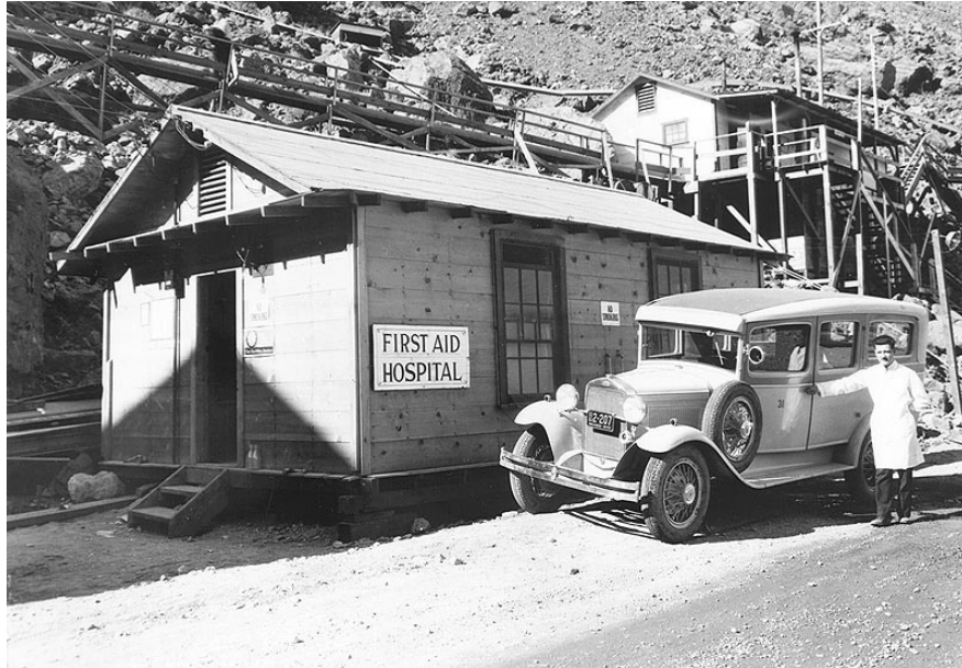
FIG. 31. One of the medical dispensaries positioned on the job site after the deaths of more than a dozen men working in the diversion tunnels without forced-air ventilation. These were equipped with a doctor, nurse, ambulance, and driver (USBR).
