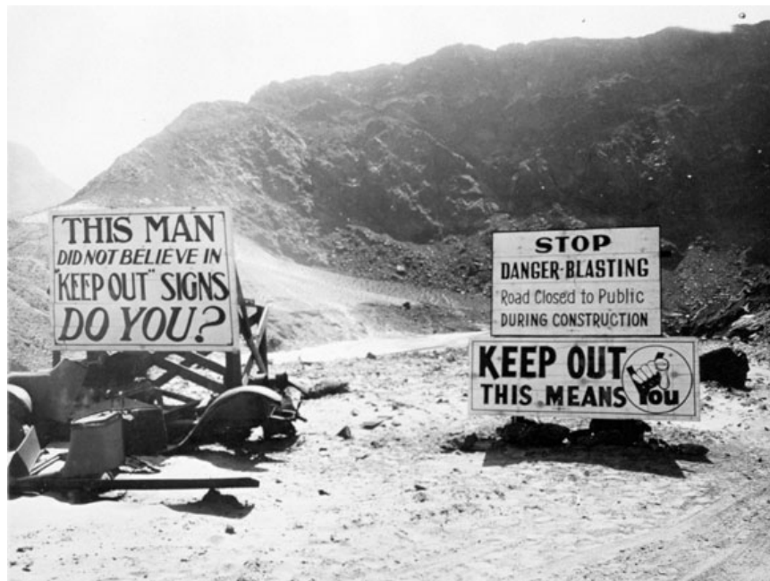
FIG. 32. As the job progressed, increasing attention was paid to safety and security after accidents or carelessness had taken the lives of workers. These signs appeared after an accident involving a driver who failed to yield to one of the between-shift blasts in 1933 (USBR).
