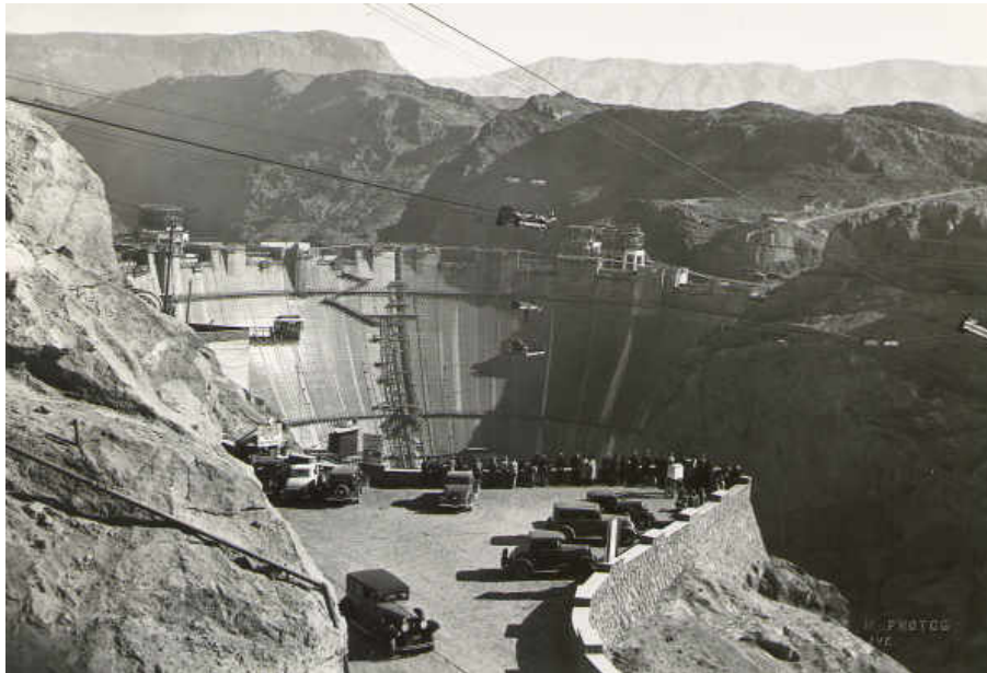
FIG. 16. “Gawkers” gather at the temporary overview at the terminus of the government highway about 3/8 mile downstream from the dam’s Nevada abutment, as seen in February 1935 (USBR).
