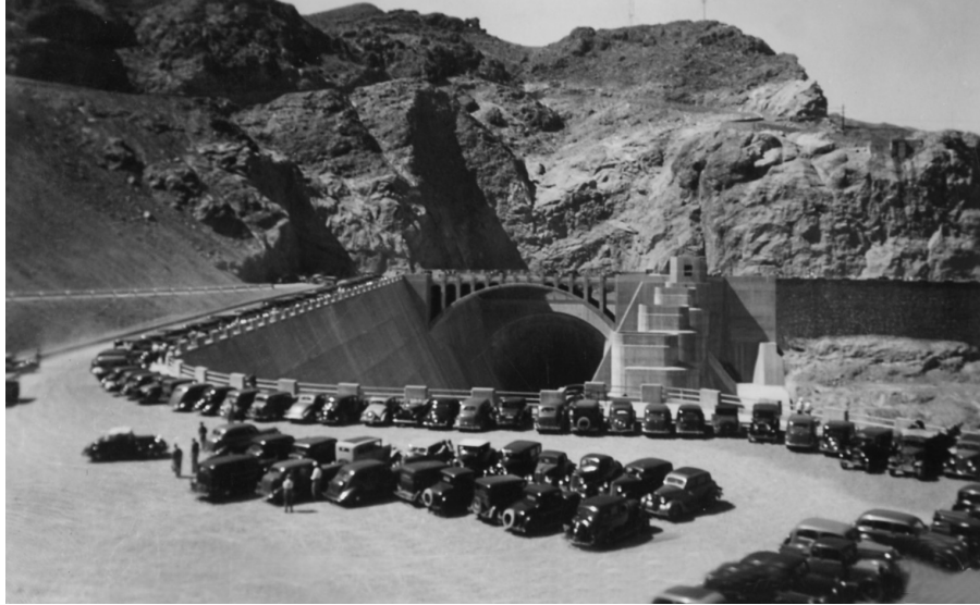
FIG. 17. Once the dam was dedicated and opened to the public the National Park Service had to cope with traffic congestion and finding suitable parking areas. This 1938 view shows the first parking lot, just upstream of the voluminous Arizona Spillway intake. Another higher lot, from which this photo was taken, was added a short while later. Visitors walked to the dam and took the public elevator down to the power house (USBR).
