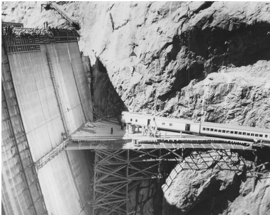
FIG. 19. Another view of the M10000 Streamliner visit in 1934, on the wooden trestle of Six Companies' low-level spur, at the Nevada abutment on the dam's upstream face (USBR).
