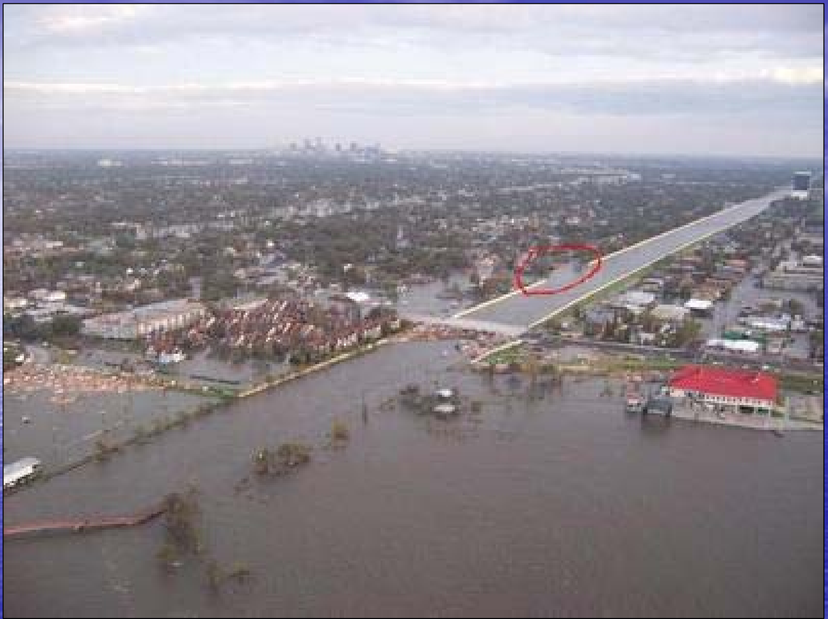
The break on the 17 th Street Canal is circled. Note debris piled up against Hammond Highway Bridge in foreground.
