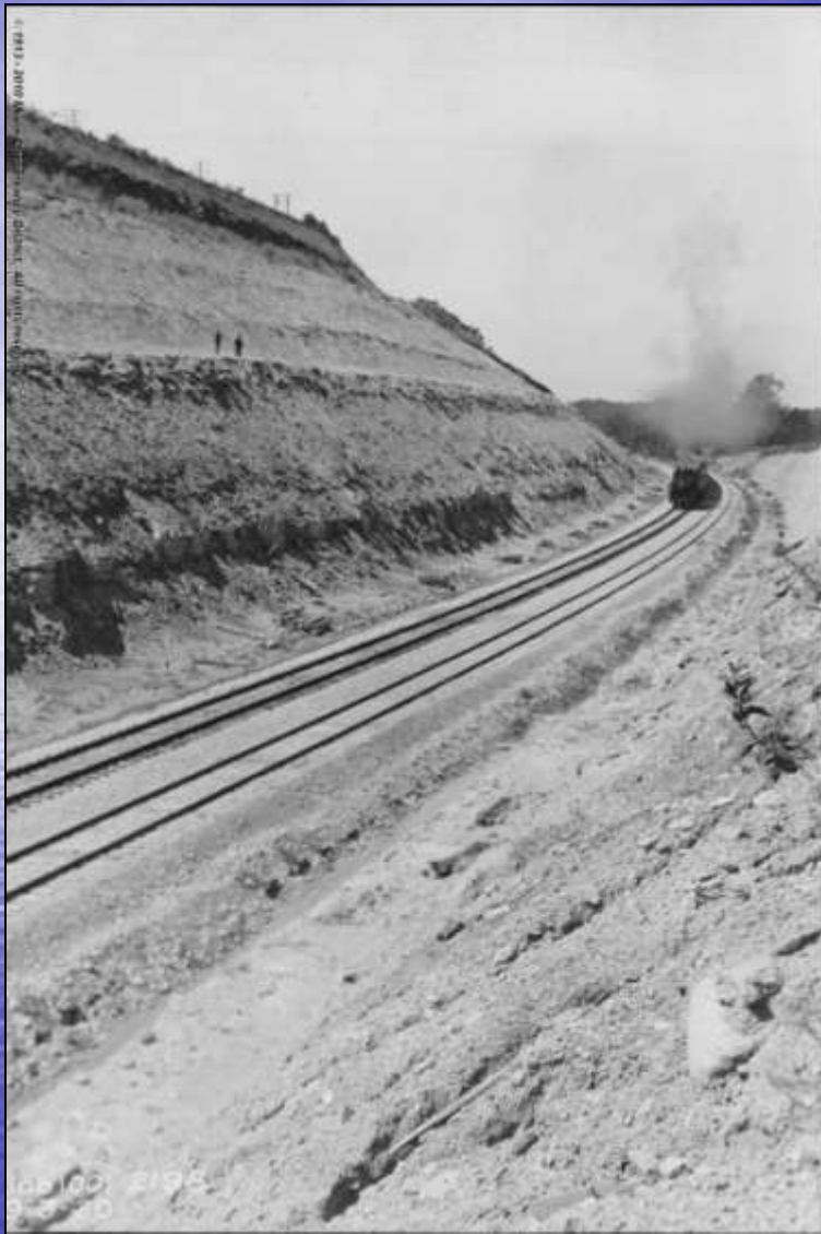
Cut for railroad relocation through Huffman Hill in September 1920. The dam's left abutment is out-of-view to the right
