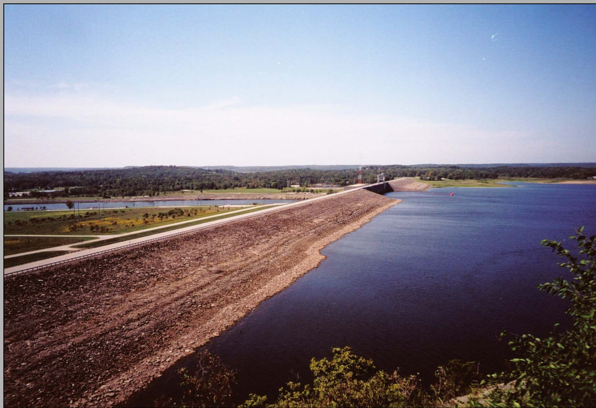
Truman Dam is an earth embankment dam similar to the proposed Meramec Dam.
