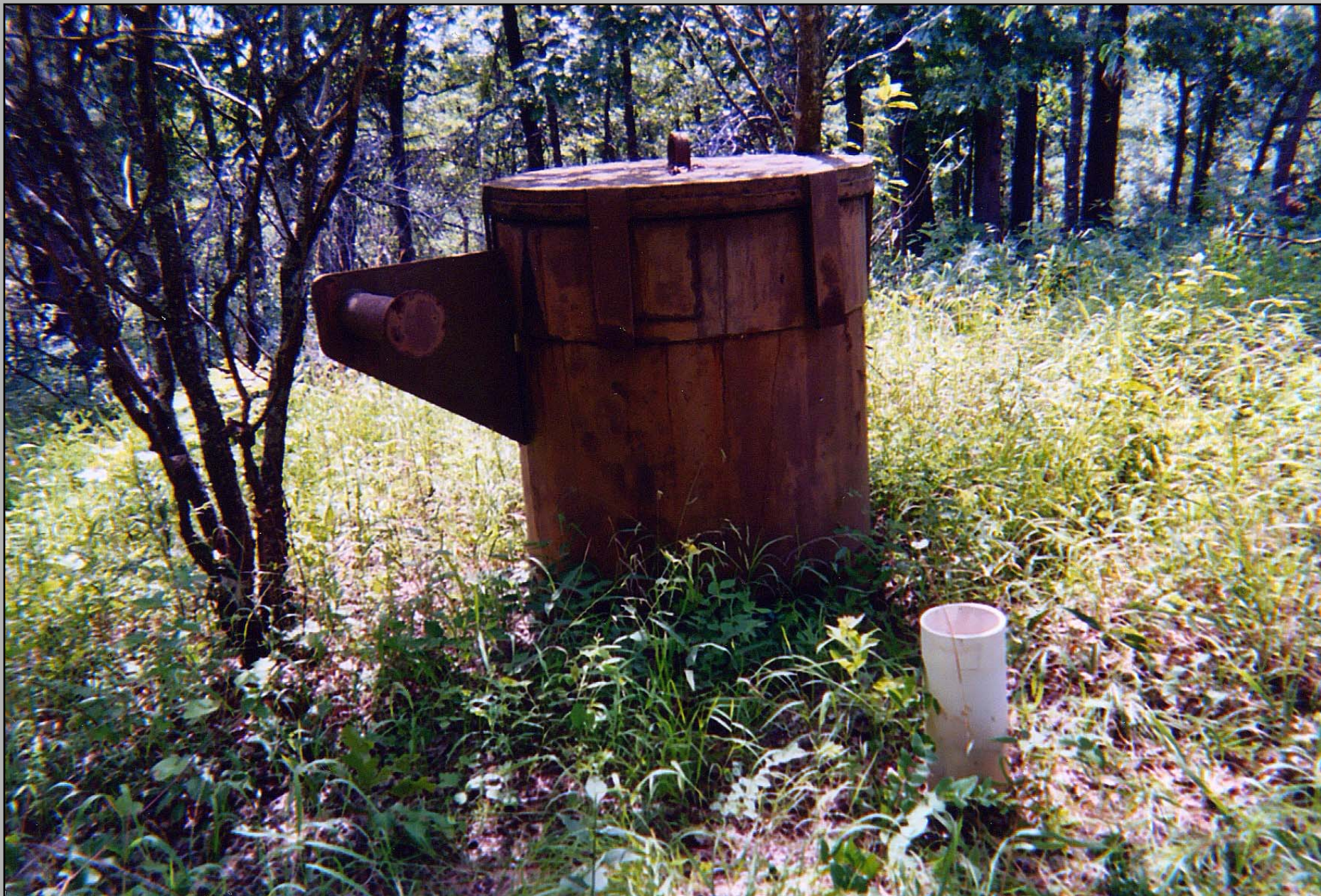
The only entrance to Moore's Cave is this 36" diameter shaft that was excavated by a calyx rig during construction for Meramec Dam.
