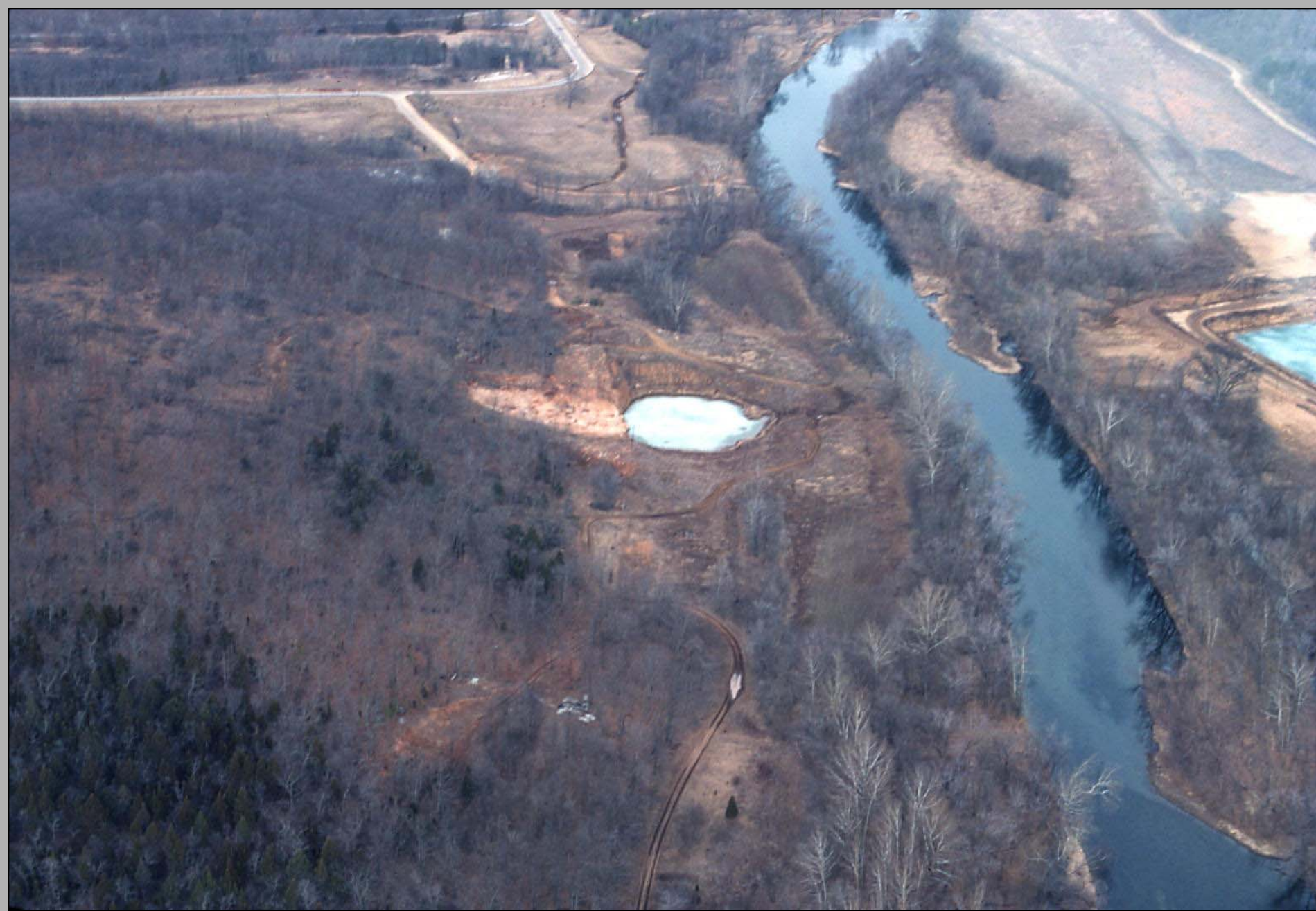
Excavations preparing dam abutments as they appeared in Feb 1977
