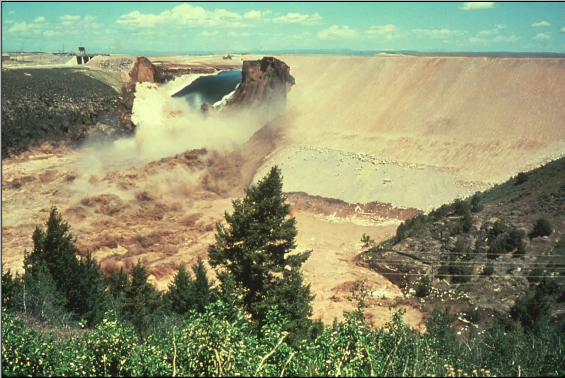
The catastrophic failure of the 350' high Teton Dam in 1976 was partly due to a poor design and construction where the abutments (sides) of the dam met the heavily fractured surrounding rock.
