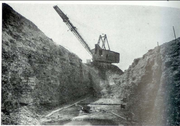
Rock excavation for outlet conduits at Englewood Dam.
