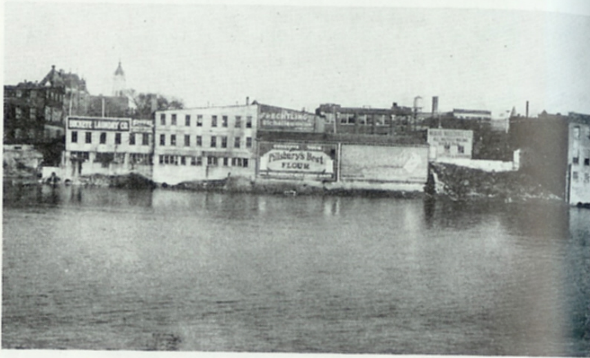
River channel at Hamilton before improvement.
