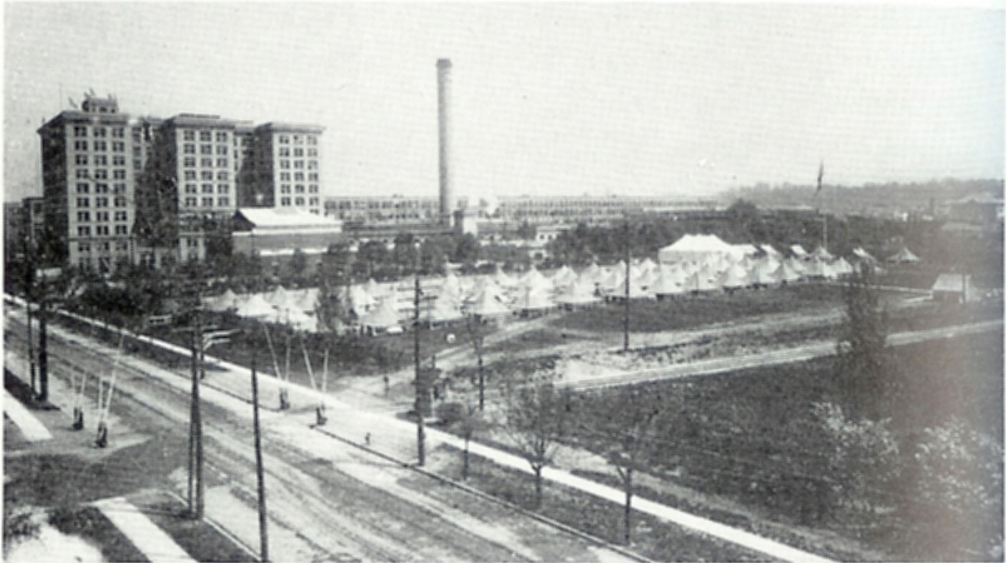
Refugee camp. N.C.R. buildings in rear.
