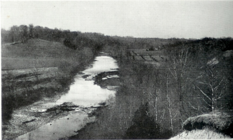
Germantown Dam site. Showing valley topography in the Miami area.
