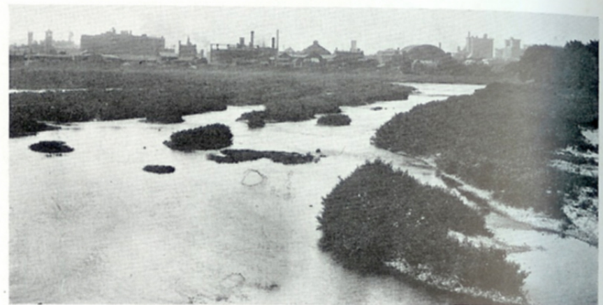
The Miami River channel at Dayton before Conservancy improvements.
