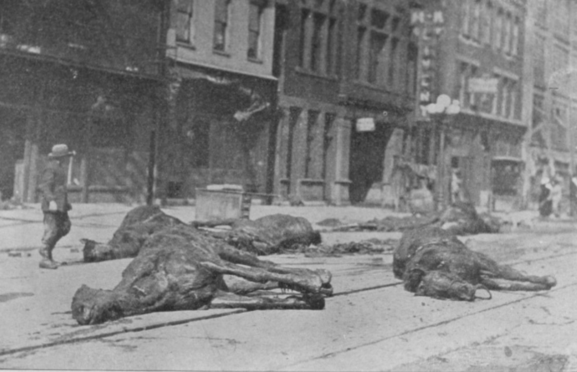
COPYRIGHT, BY UNDERWOOD & UNDERWOOD, N. Y. STREET IN DAYTON AFTER THE FLOOD RECEDED SCENE IN THE BUSINESS SECTION, SHOWING DEAD HORSES DROWNED IN THE FLOOD. HORSES WERE DROWNED IN THEIR STALLS IN MANY CITIES.
